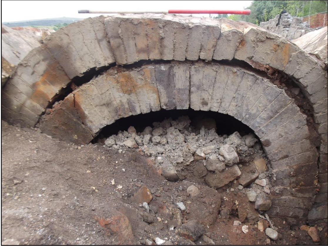
Plate 94. North Coppée coke oven flue complex, mouth of the western flue (flue 2458) opening into flue junction 2464. View to west.
