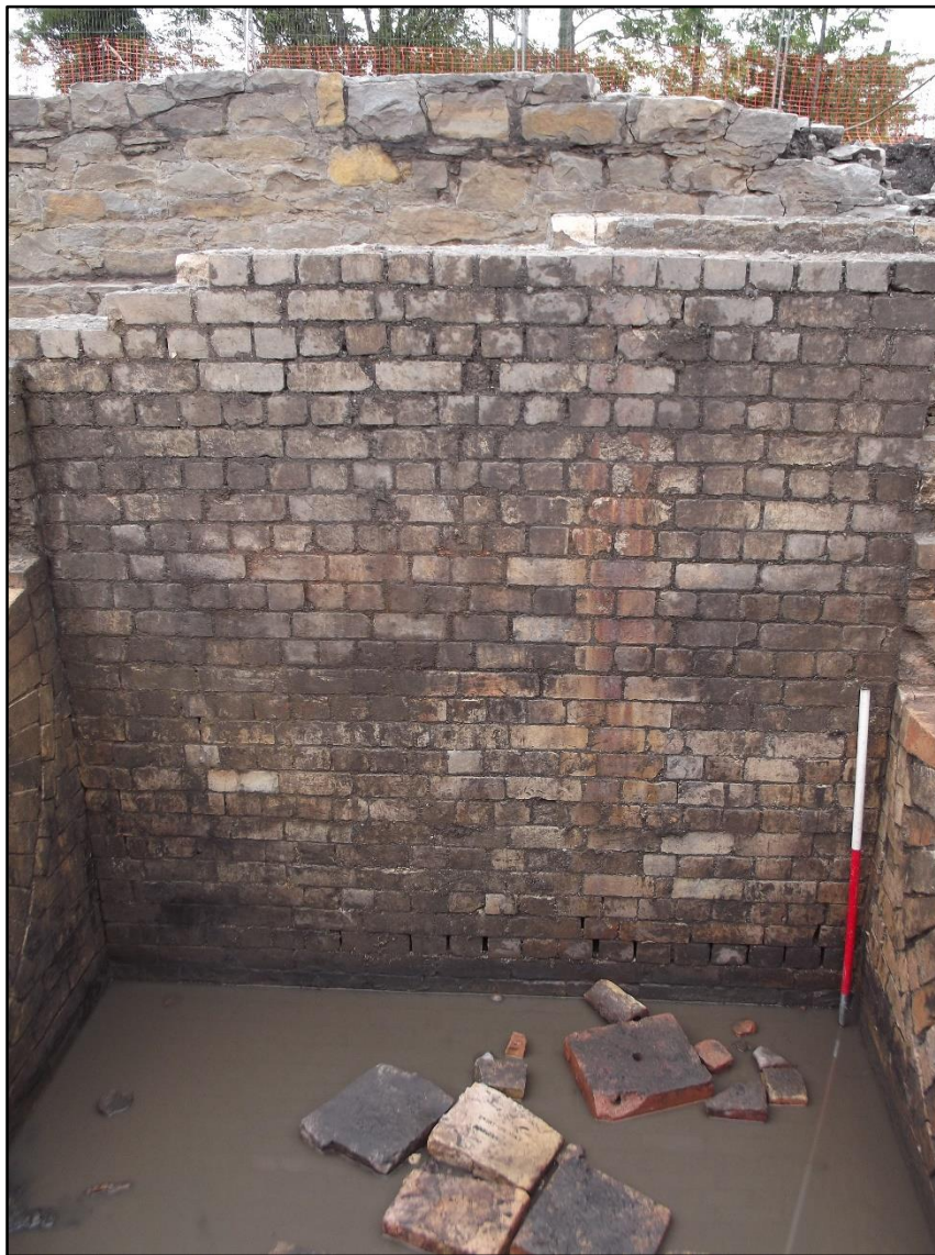
Plate 90. North Coppée coke oven complex, north wall of chimney base 2132. The structures just visible to left and right are the mouths of main gas flue 2448. View to north.
