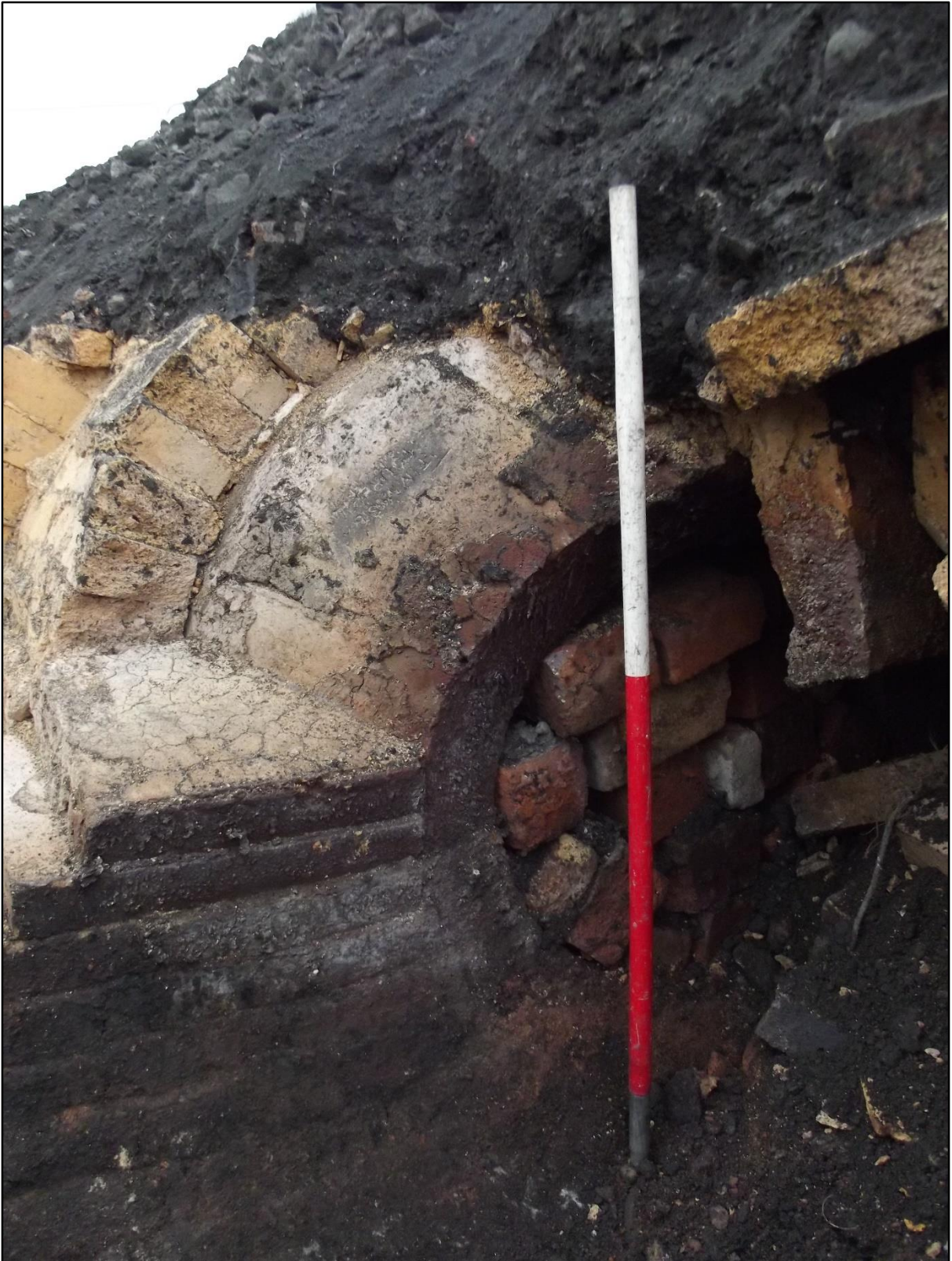
Plate 123. South Coppée coke oven flue complex, crude blocking visible at the junction of flues 2555 and 2526. This blocking may be contemporary with the modifications evident in the chimney base chamber (see below). View to north east.
