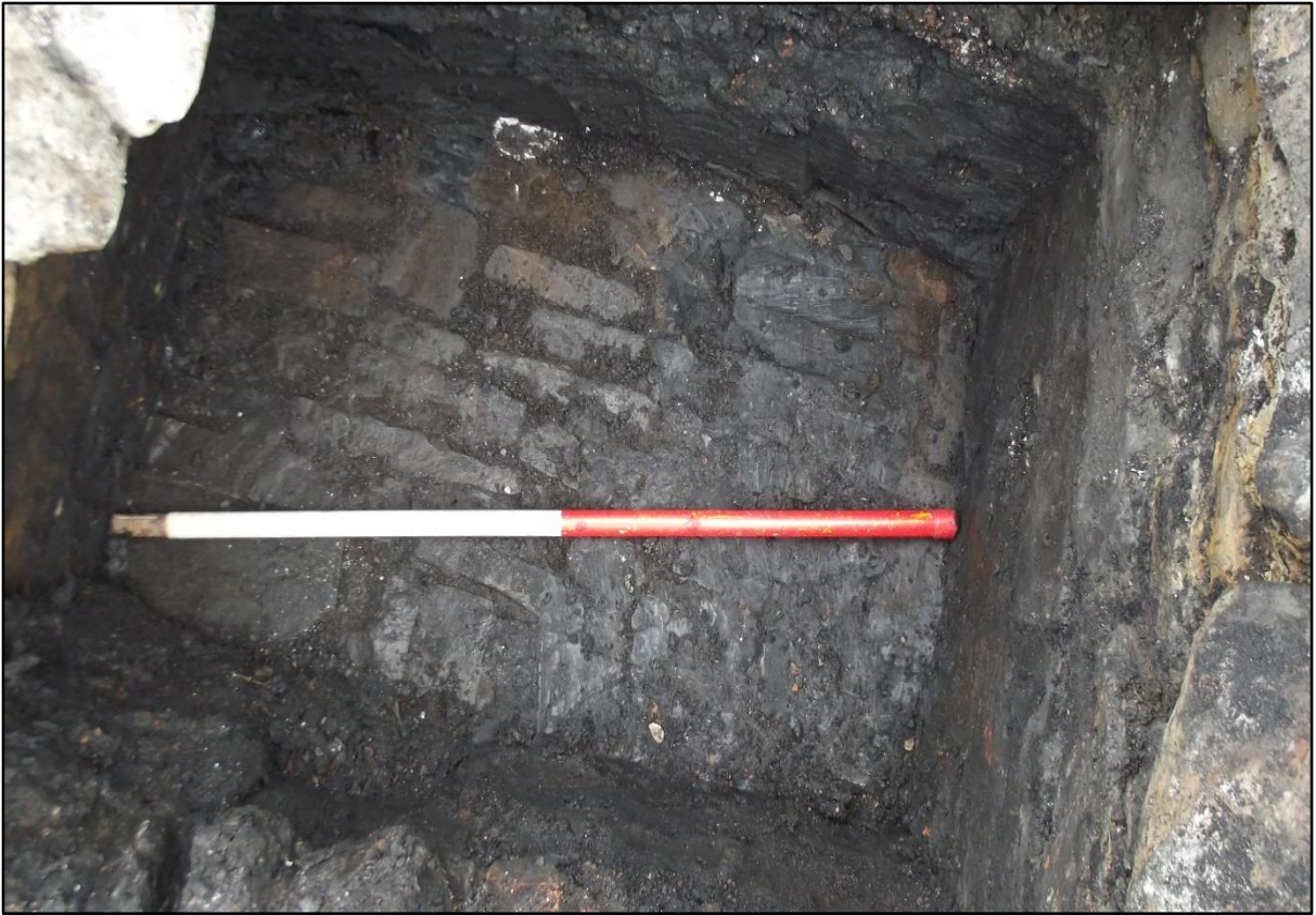
Plate 30. Coke yard area, stone floor of culvert 2295. Note the traces of clay on the upper stone courses.
