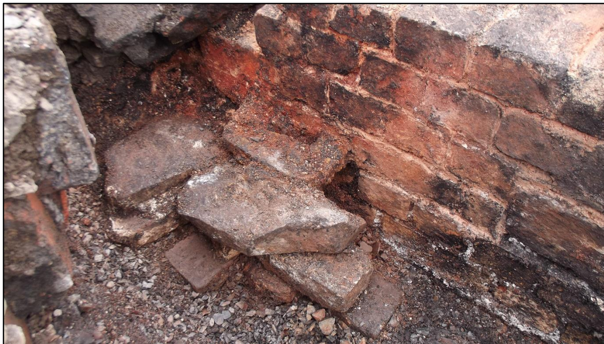
Plate 20. Close up of the 'D' shaped stay associated with the door fittings on the Thomas ovens.
