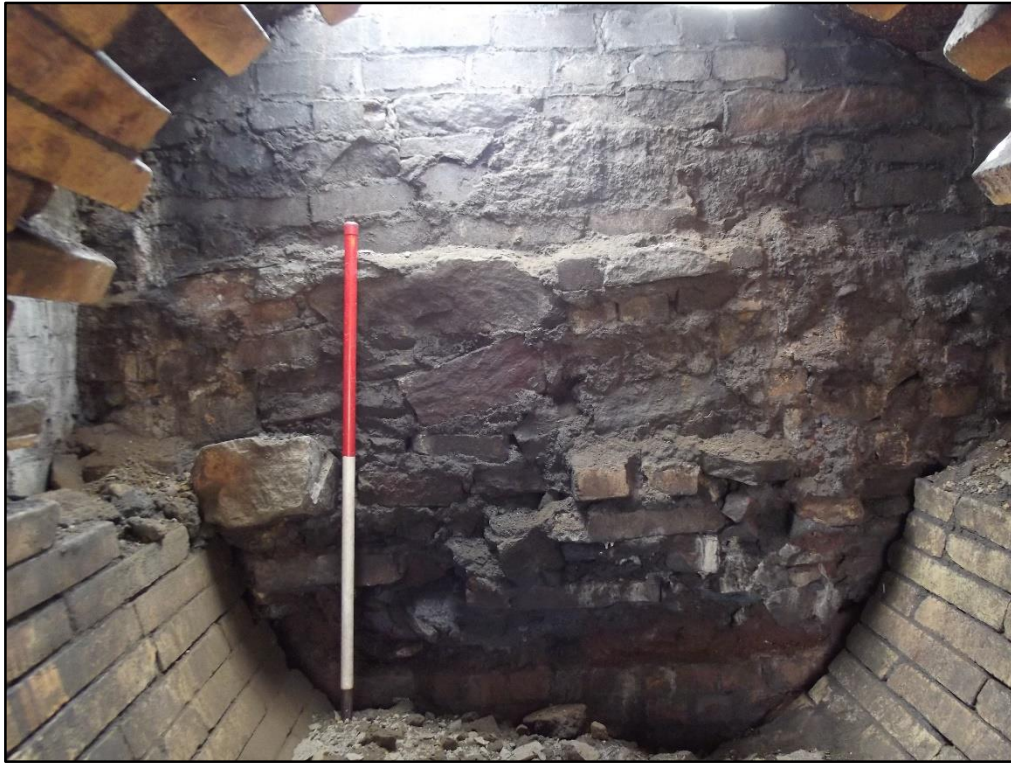
Plate 85. North Coppée coke oven flue complex, view of the interior of the western end of main gas flue 2448 showing the lower half of the flue abutting wall 2433. View to west.
