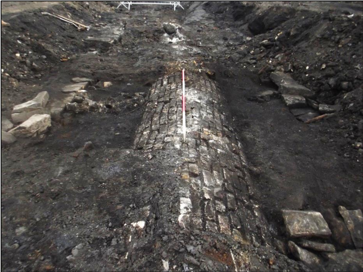
Plate 8. Culvert 2003 on removal of the capping. Note its position within the channel of the canal. View to south.
