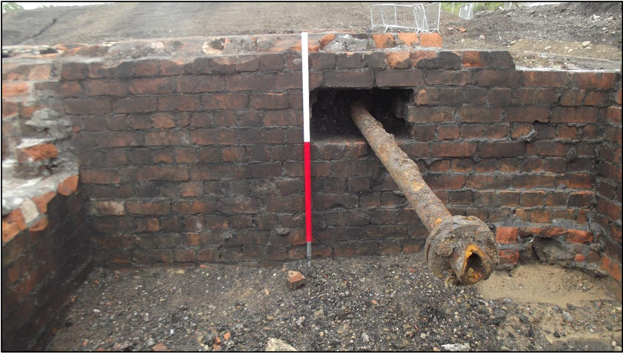
Plate 55. High pressure steam or water pipe 2044. This pipe probably helped to supply power or water for the Sheppard Feldspar washer located west of the settling tank and was one of the few remaining elements of it to have survived.
