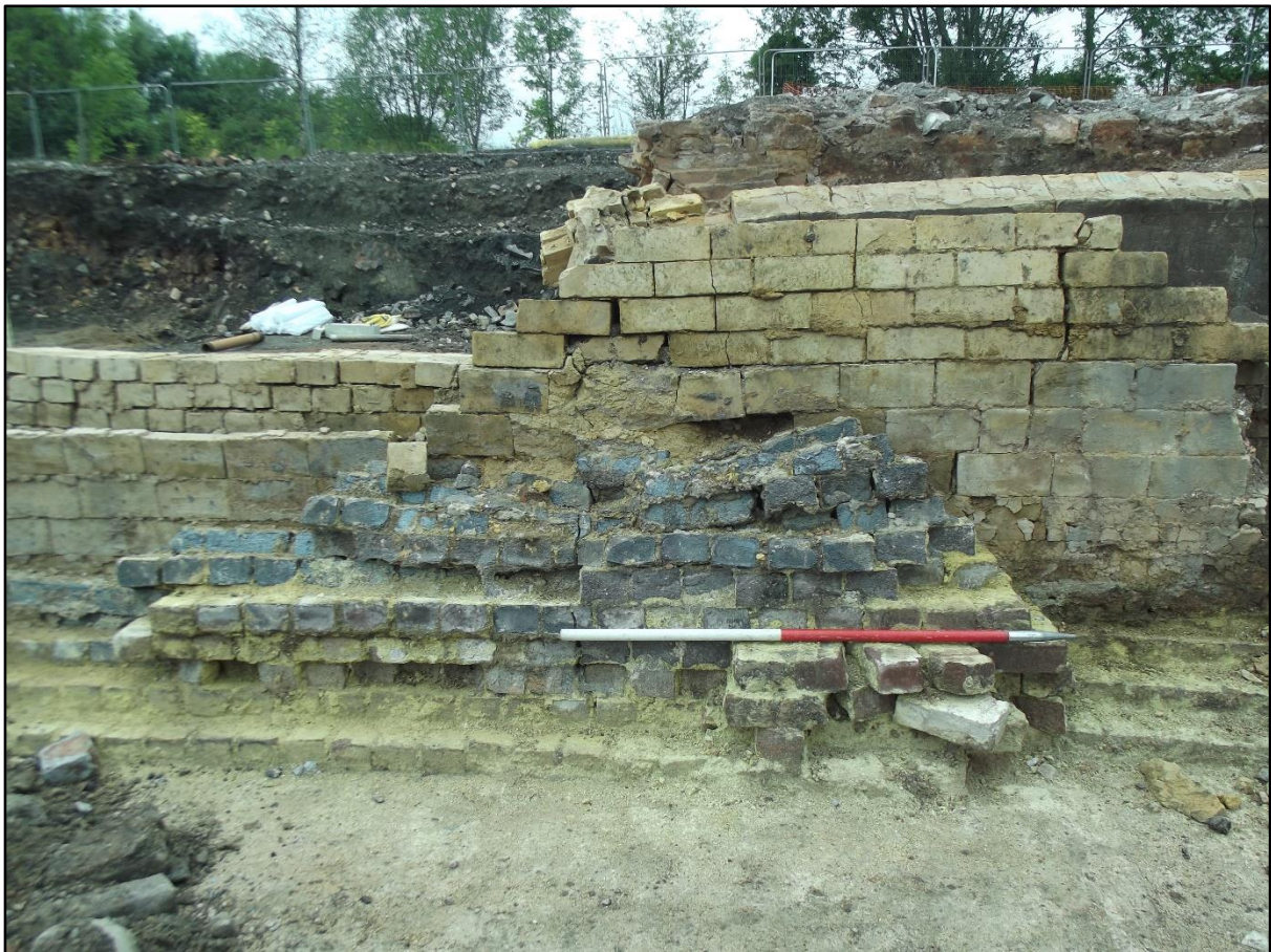
Plate 78. North Coppée coke oven battery, the south wall of the main gas flue (wall 2436) to the rear, and feature 2508, with a ranging rod resting on it. feature 2508 may, in fact have been the only surviving portion of the walls of the transverse flues for the ovens. View to north.
