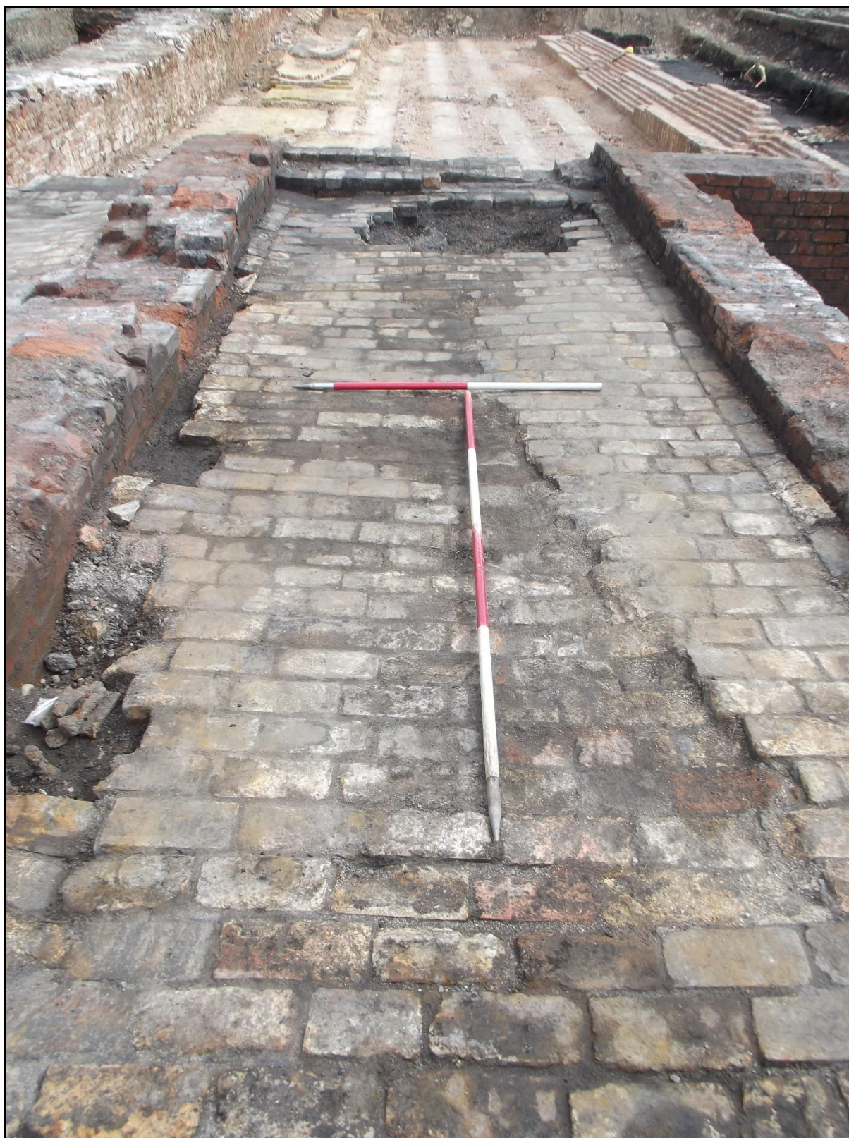
Plate 64. North Coppée coke oven battery. Floor surface 2219 looking east to the remains of the coke ovens. This floor is believed to be associated with the transportation system for moving processed coal to the top of the Coppée coke ovens. Note the extensive wear to the surface of the bricks.
