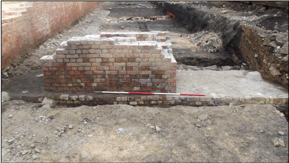
Plate 136. North Coppée coke oven battery, chamber 2309 and the capping over the canal. Note that these features have cut the construction cut for the south retaining wall of the coke ovens (construction cut 2300).
