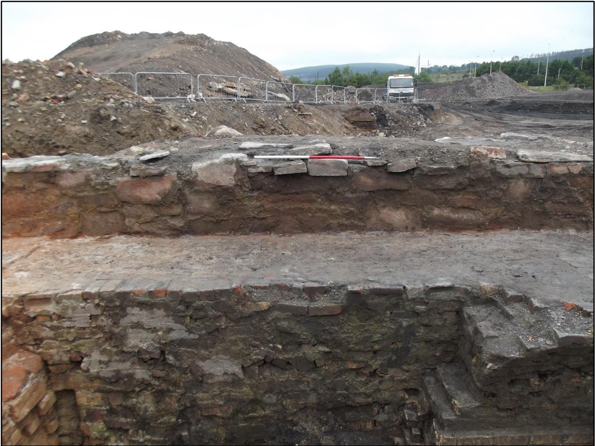
Plate 80. North Coppée oven flue complex, north elevation of wall 2437. Note the absence of a stepped foundation. Brick floor 2481 is visible, as is part of a chamber forming part of chimney 2464. View to south.
