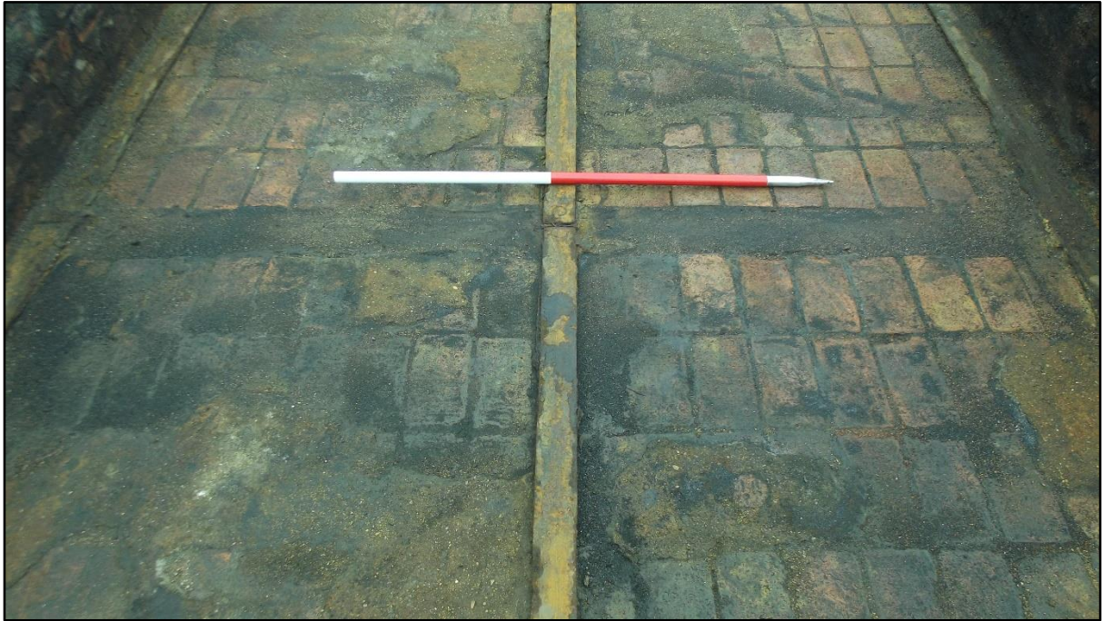
Plate 53. Closer view of the iron strips on the base of the settling chamber. They had been secured to the timber sleepers by round flathead nails. Scale is 1m.
