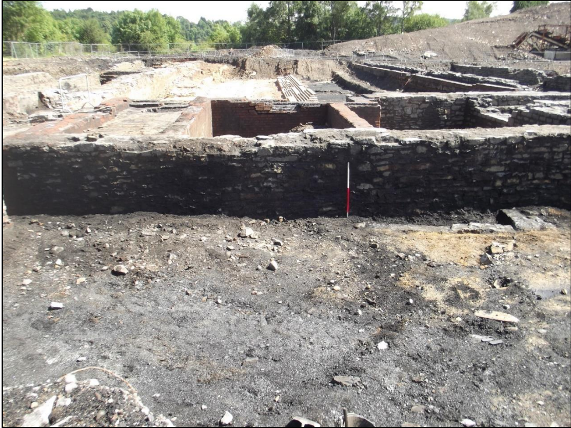
Plate 60. Western elevation of the Phase 3b of the coal storage bunker (wall 2213). Also visible are the brick wall partitions inside the structure to create the bunkers. View to east.
