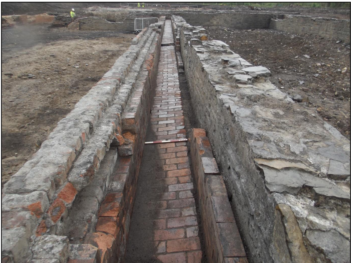
Plate 114. South Coppée coke battery coke bench, trough 2201 looking west. Note that the gap that opened between the trough and wall had been partially filled with brickwork, suggesting that subsidence had been an issue during the operational lifetime of the coke bench.
