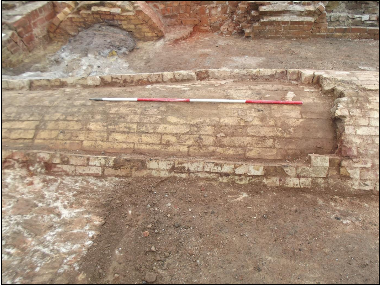
Plate 83. North Coppée oven gas flues, roof of the main gas flue 2448 showing the outer skin of standard refractory brick and the outer surface of the specialist wedge shaped brick that formed the flue itself. Scale is 2m. View to south.
