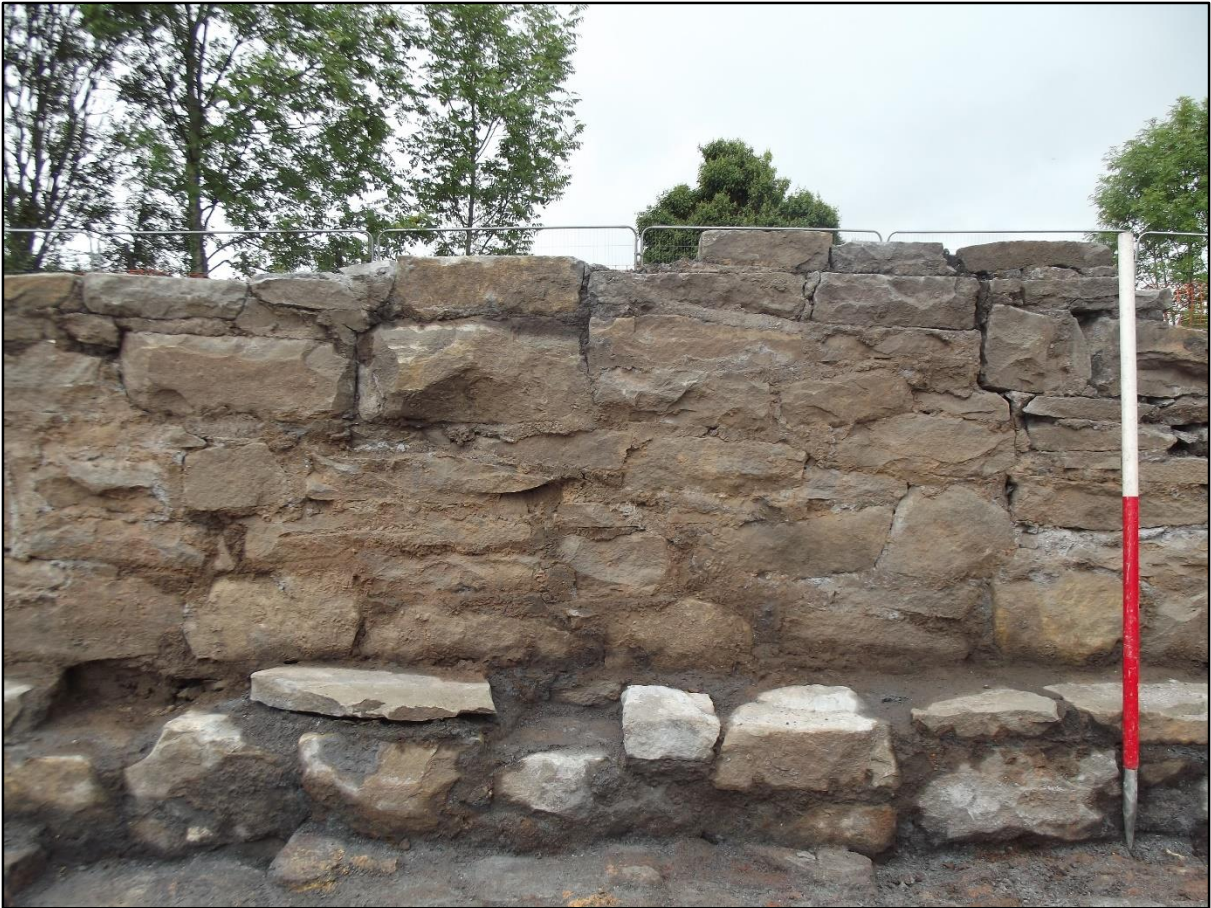
Plate 79. North Coppée coke oven flue complex, south elevation of wall 2442 showing stepped foundation. View to north.
