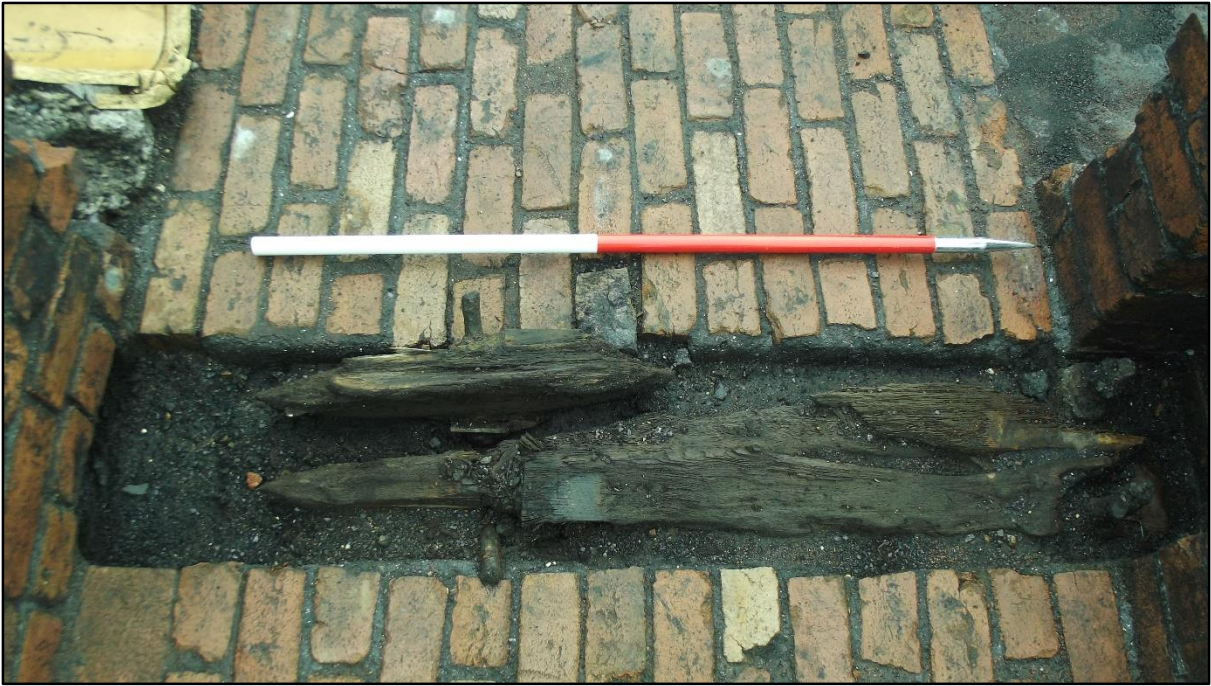
Plate 59. Remains of timber sleeper 2107 set within floor 2072. Scale is 1m. Note the shallow recess beneath the wall on the left of the photograph which permitted insertion of one side of the sleeper; the opposite end could then be dropped into place using the larger recess in the opposite wall.
