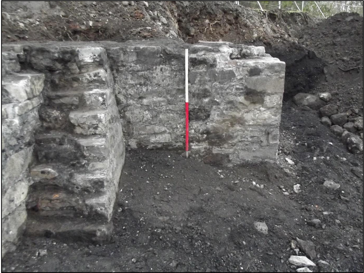
Plate 18. Smithy area, L shaped structure, showing the batter on the steps and the better quality stone quoins to the right of the image. View to east.
