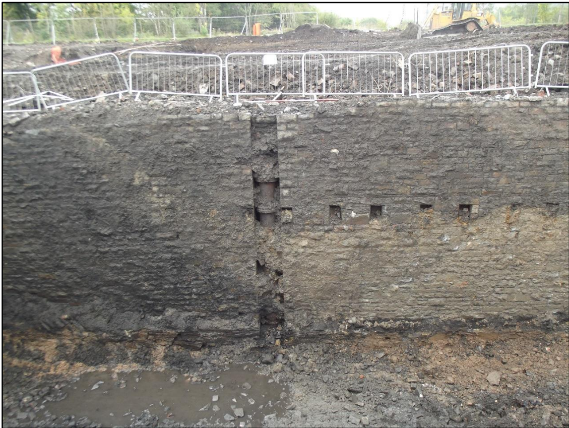
Plate 128. The vertically mounted iron pipe set within the recess in the north coke bin wall. View to north. Note also the smaller recesses fitted with iron box inserts, which probably supported a false floor within the coke bin area.
