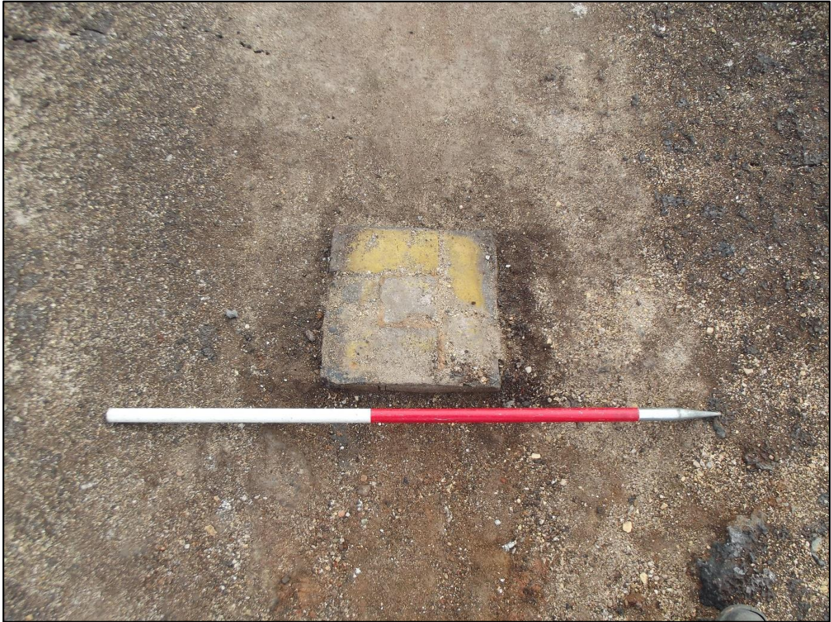
Plate 71. North Coppée coke oven battery, one of the two surviving pillar bases in the vitrified surface of the main gas flue. Scale divisions are 0.5m
