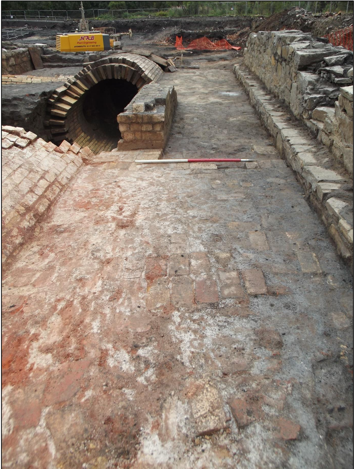
Plate 81. North Coppée coke oven flue complex, view of floor surface 2446 that formed the north side of the channel for the main gas flue in this area. Note the gas flue to the left and wall 2443 to the right. View to west.
