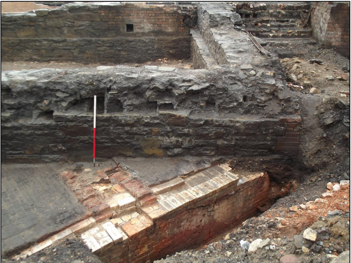
Plate 27. North side of the Thomas ovens beneath the later Coppée coke ovens. View to south.
