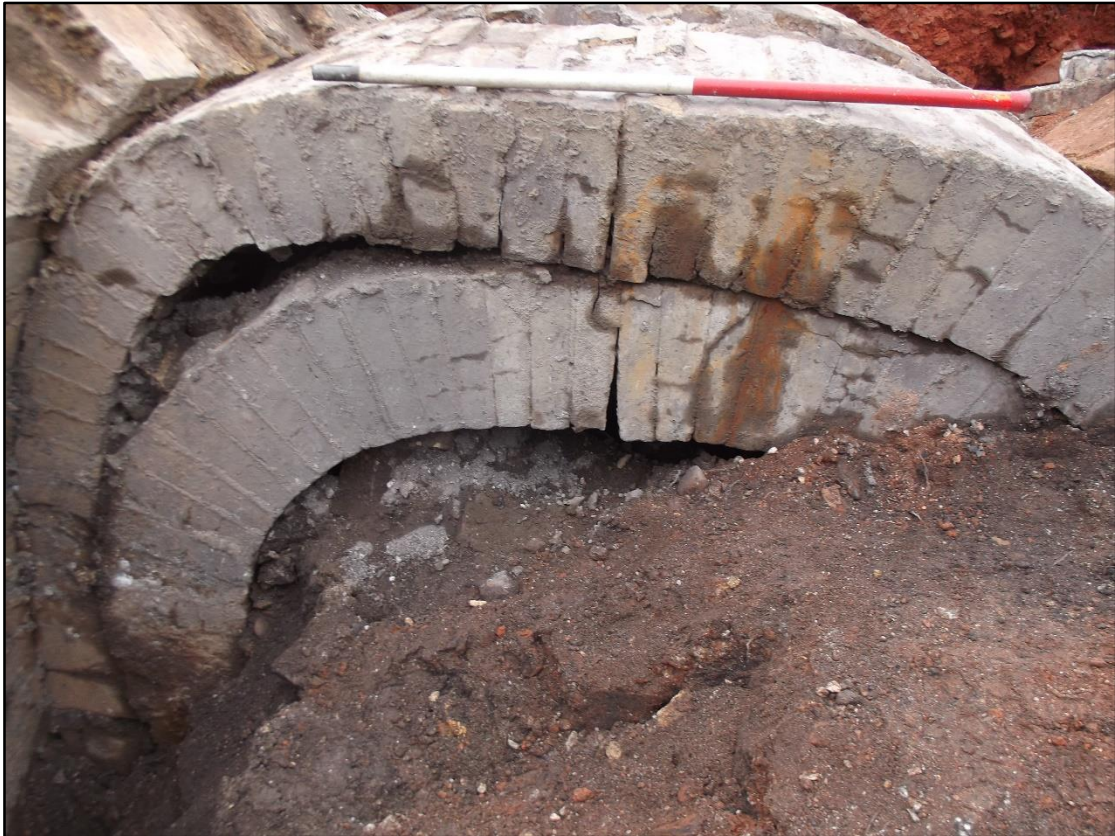
Plate 95. North Coppée coke oven flue complex, eastern flued mouth 2456 opening into flue junction 2464. View to east.
