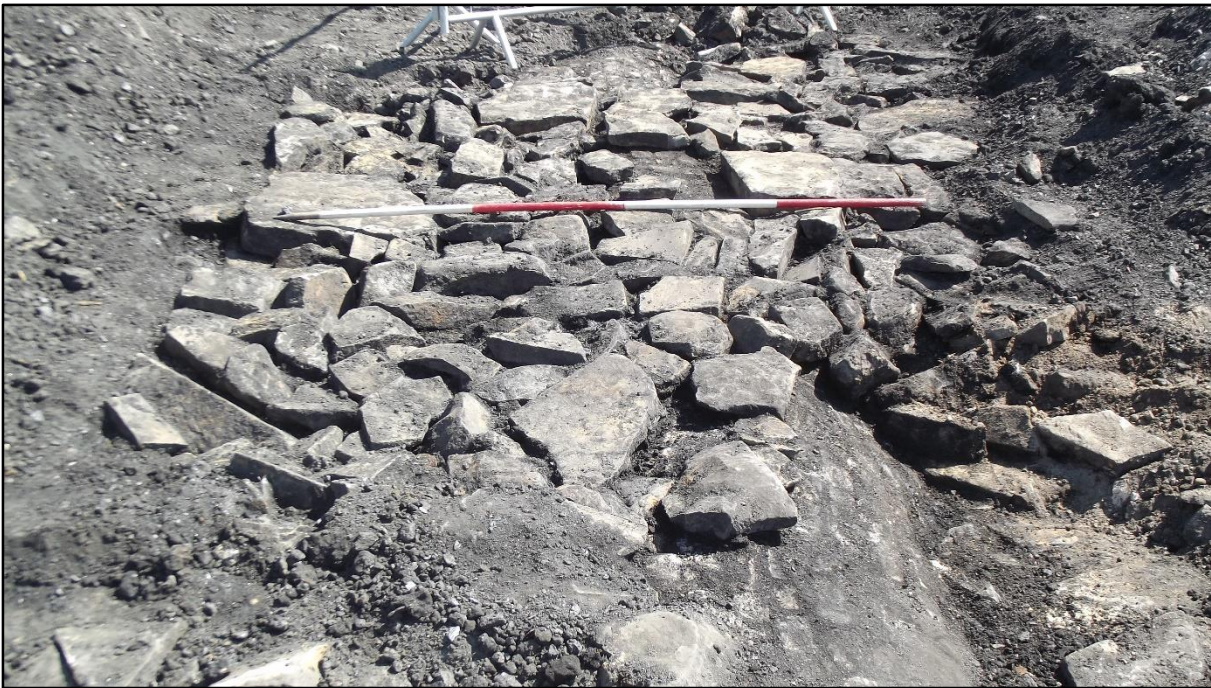
Plate 7. Stone capping 2002 which had been laid over the culvert contained by the canal. It is likely this had been placed both to level the area and protect the underlying culvert, the arch of which is just visible in the bottom right quadrant of the photograph.
