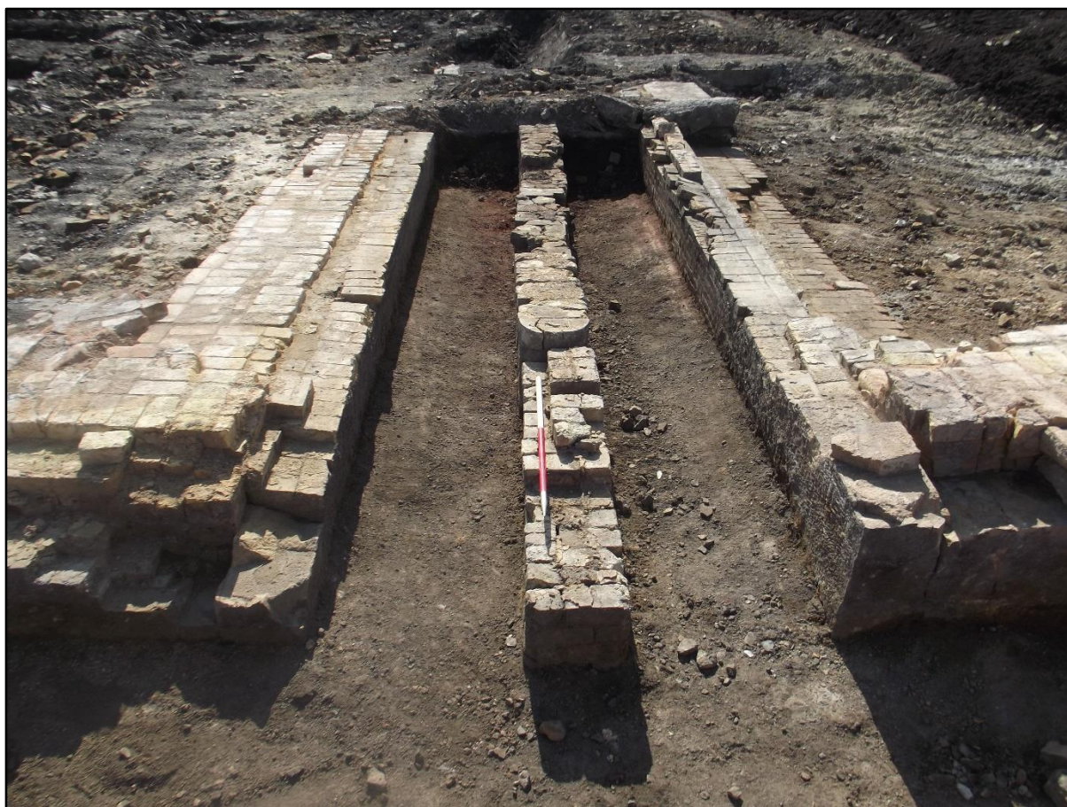
Plate 120. South Coppée coke oven main gas flue, spur to flue 2012 showing the supporting partition walls 2280 (nearest camera) and 2281. View to south.
