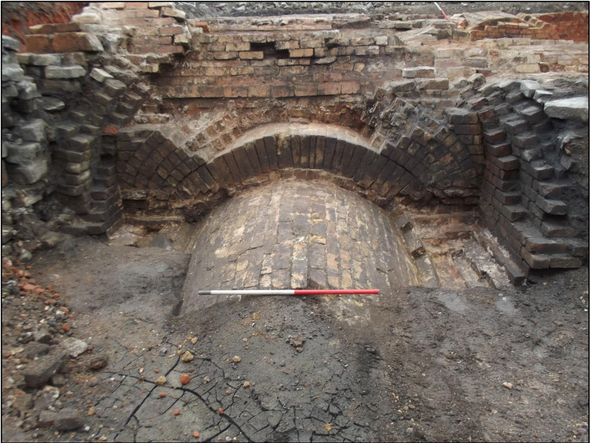
Plate 96. North Coppée coke oven flue complex, rear view of flue 2459 showing the reinforced collar of the flue and elements of the relieving arch on either side. View to south.
