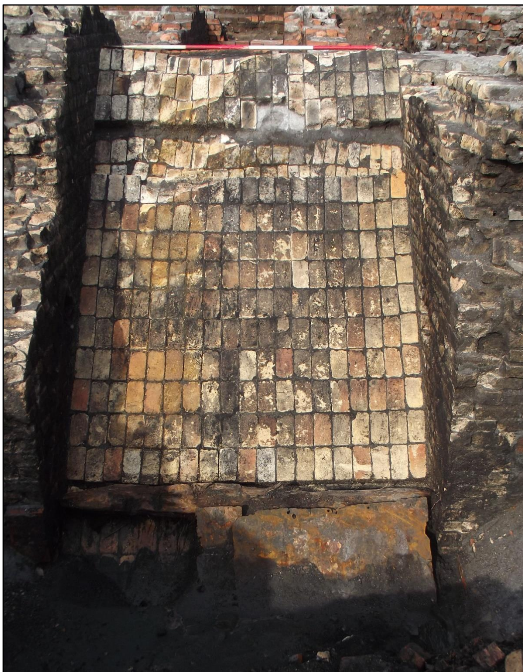
Plate 43. The western chute 2063 for the Carr's disintegrator elevator. View to west.
