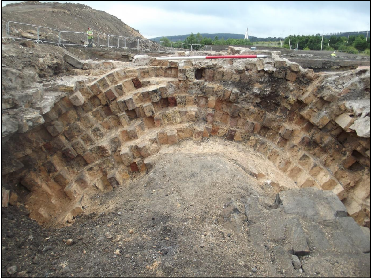
Plate 108. North Coppée oven gas flue system, brick reinforcing collar above the mouth of flue 2338/2432. The grey brickwork in the foreground is part of collapsed relieving arch 2391. View to south.
