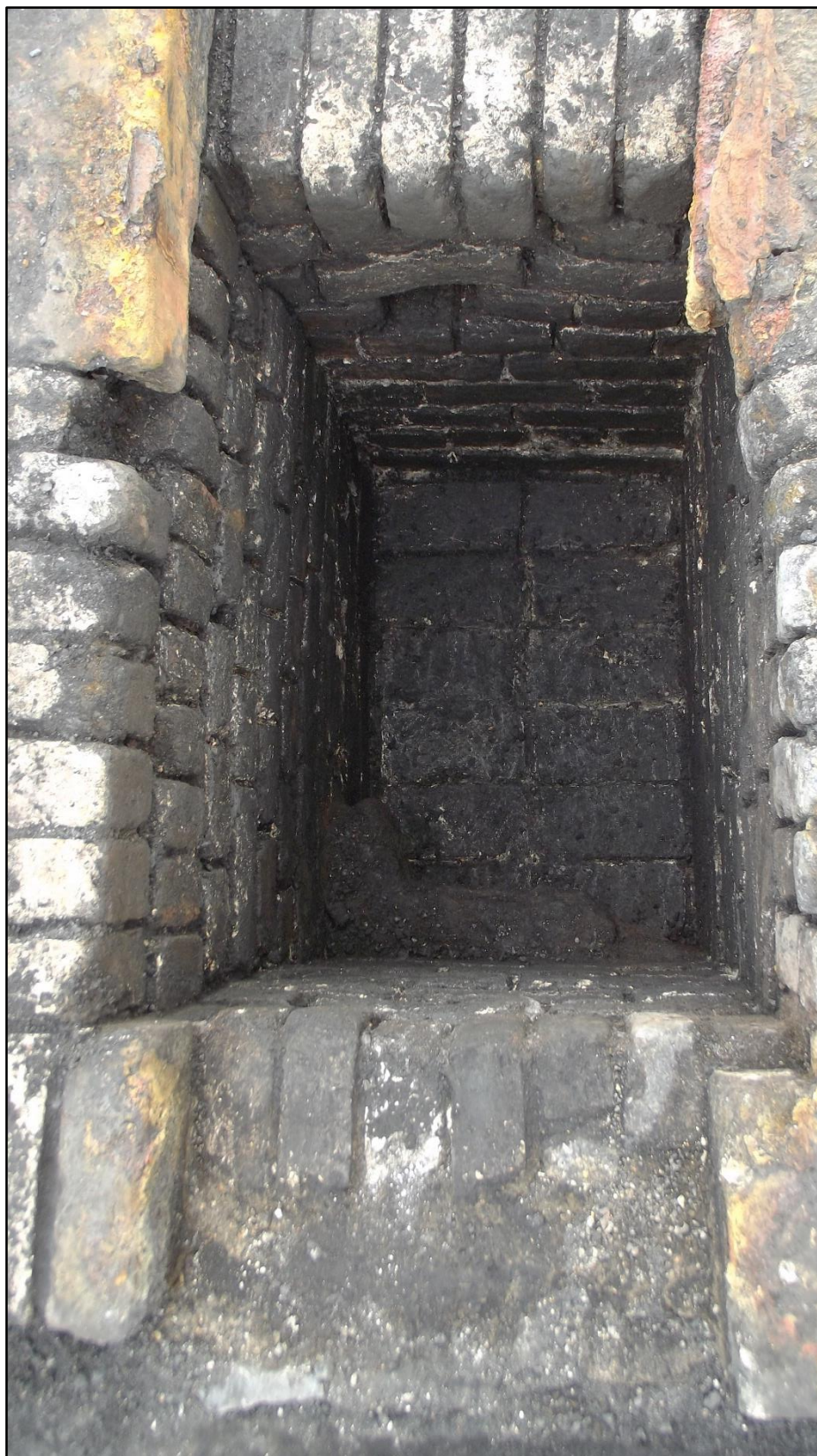
Plate 15. Interior of brick chamber 2297 showing the drain in the south west face and the floor.
