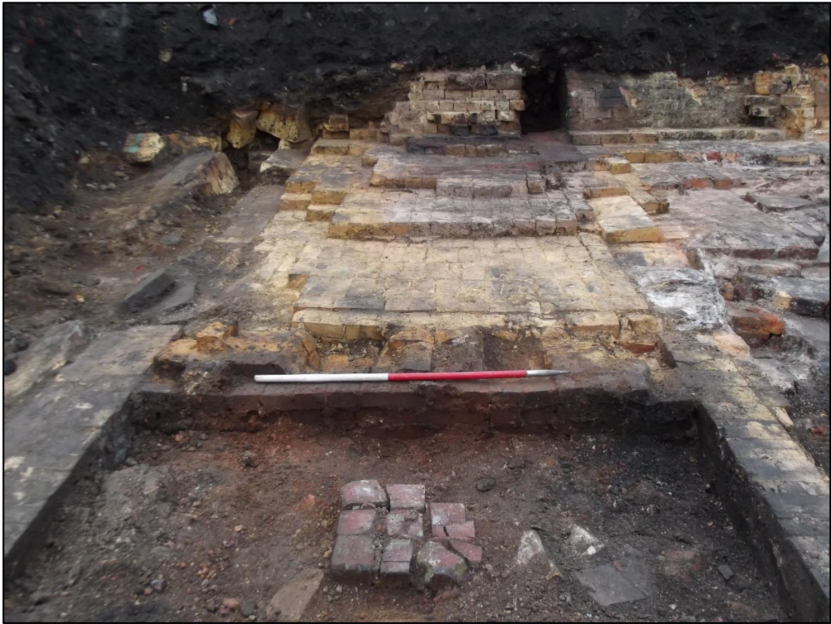
Plate 121. South coke oven flue complex, eastern terminal end of main gas flue 2012 showing one of the square pillar bases that supported the roof and the brick bay grouping beyond. The level of vitrification was greater here than for the northern flue. View to east.
