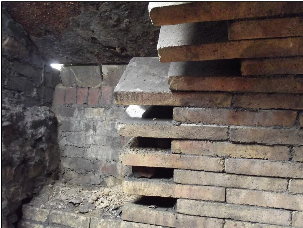
Plate 86. North Coppée coke oven gas flue complex, view of the unfinished western terminal of flue 2448. View to north west.
