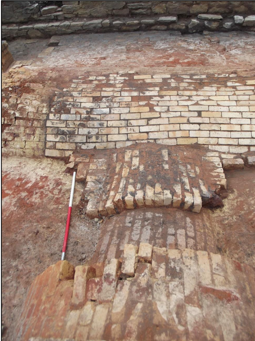
Plate 89. North Coppée coke oven flue complex, repair or insert to the roof of the main gas flue 2448. The repair may have been intended to remedy a collapse of secondary flue 2447, which is visible at the bottom of the image. View to north.
