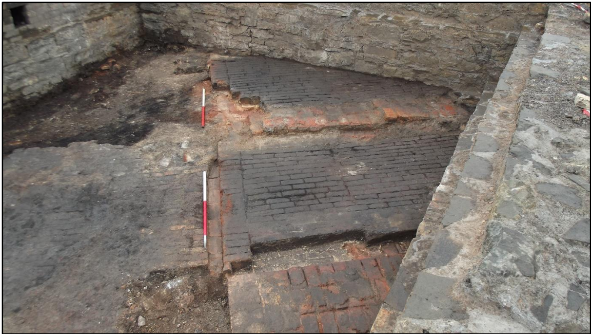
Plate 22. View to the south west of the internal floor surfaces of the Thomas ovens. The internal divisions are marked by the absence of bricks whilst the coking bench is the damaged brick surface to the left of the ranging rods. Slot 2366, a recess for the coke oven doors can be seen immediately right of the ranging rods. The upstanding walls are the remains of the later Coppée oven which was constructed in the 1880s.
