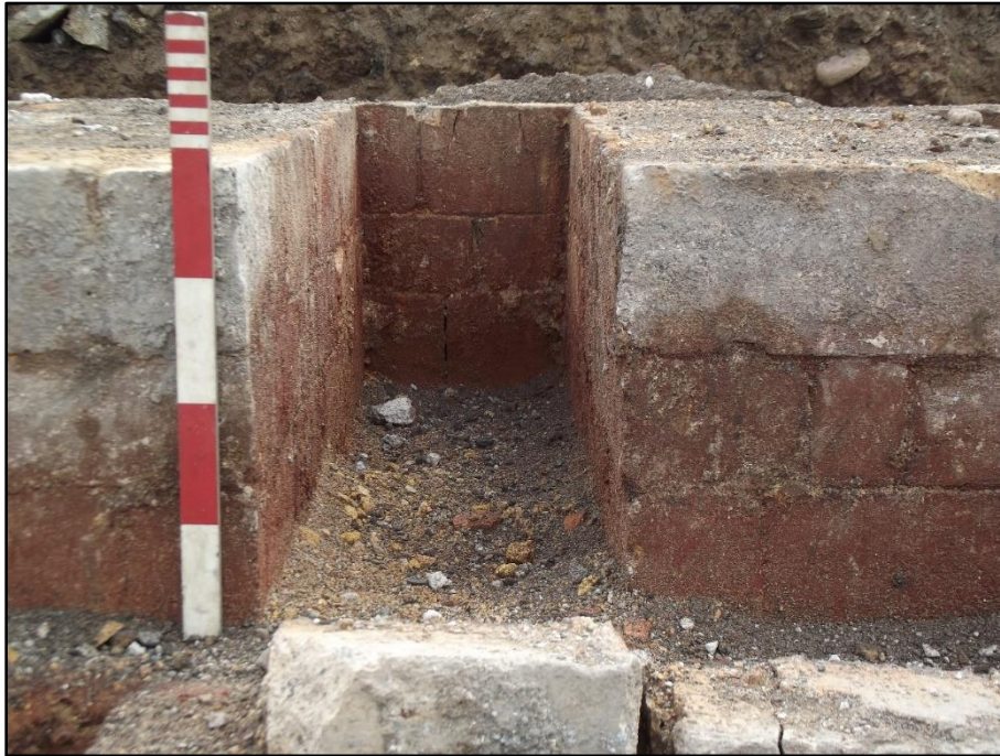
Plate 103. Close up view of the construction of one of the bays forming part of group 2468, part of the north coke oven battery. Note the reddened appearance caused by intense heat.
