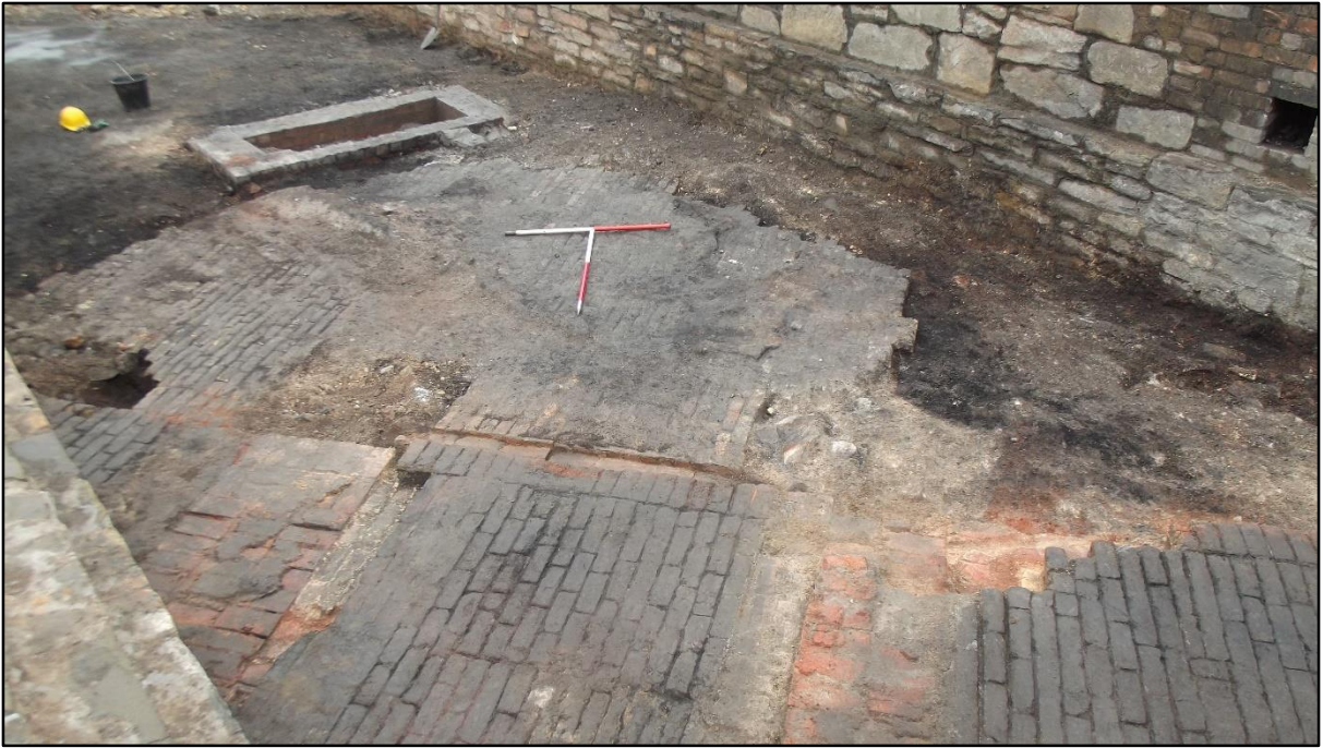
Plate 26. Interior floors of the Thomas ovens and coke bench showing the relationship with later brick chamber 2341. View to east.
