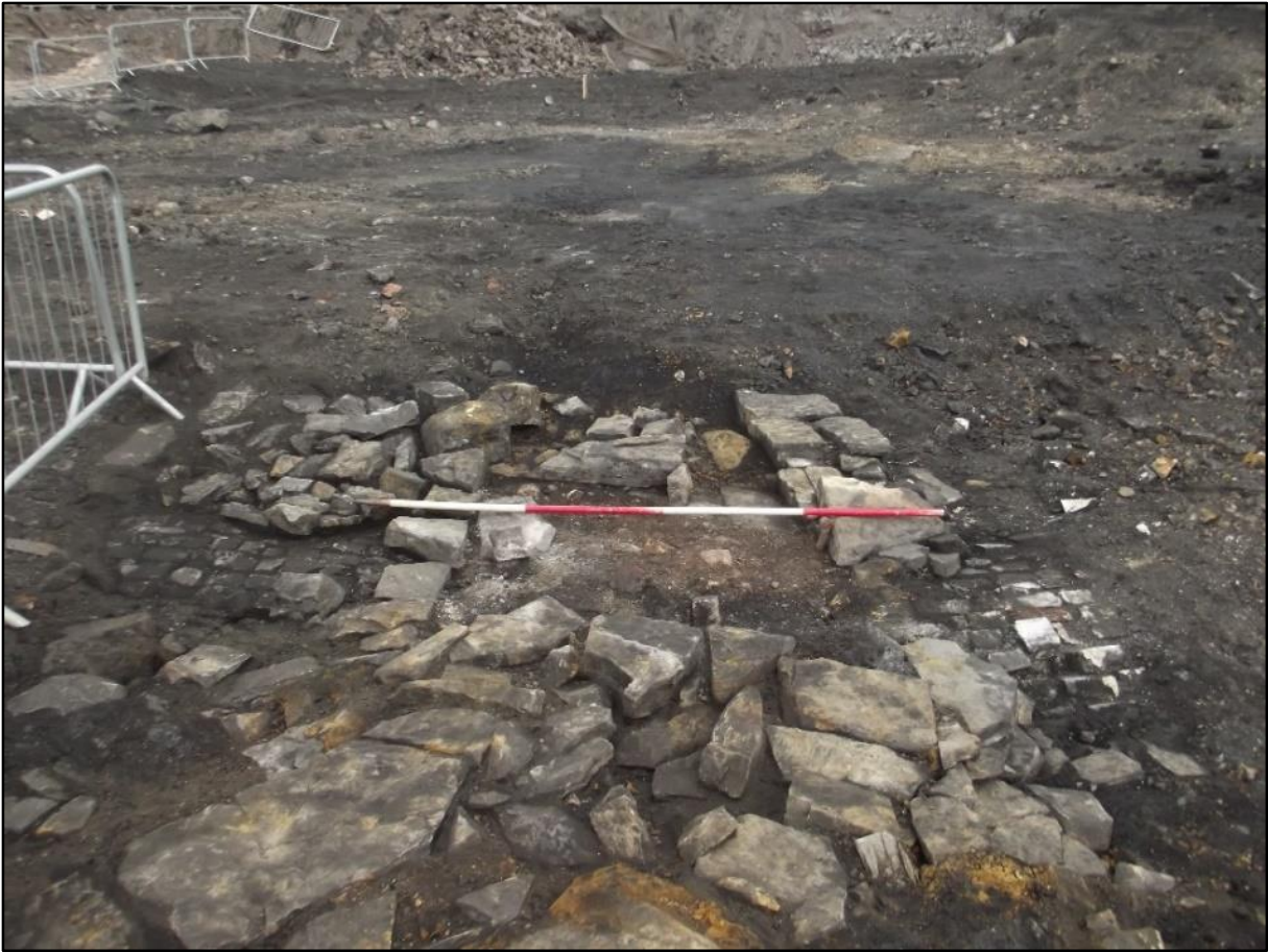
Plate 9. Crossing point 2021 sited over culvert 2003. View to north east.
