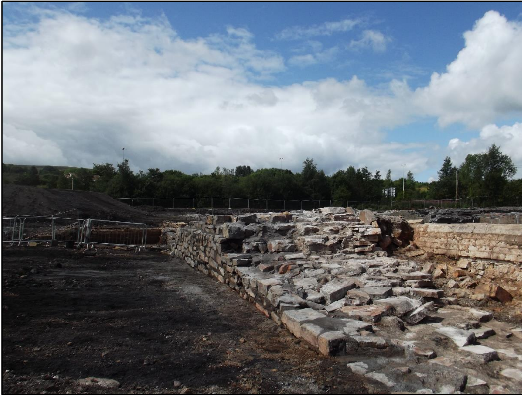
Plate 118. South Coppée coke oven coke rammer walls, oblique view of the rammer walls and the main gas flue to the rear. This image provides an indicator of the combined width of the wall in this location, which was in excess of 2m. View to north west.
