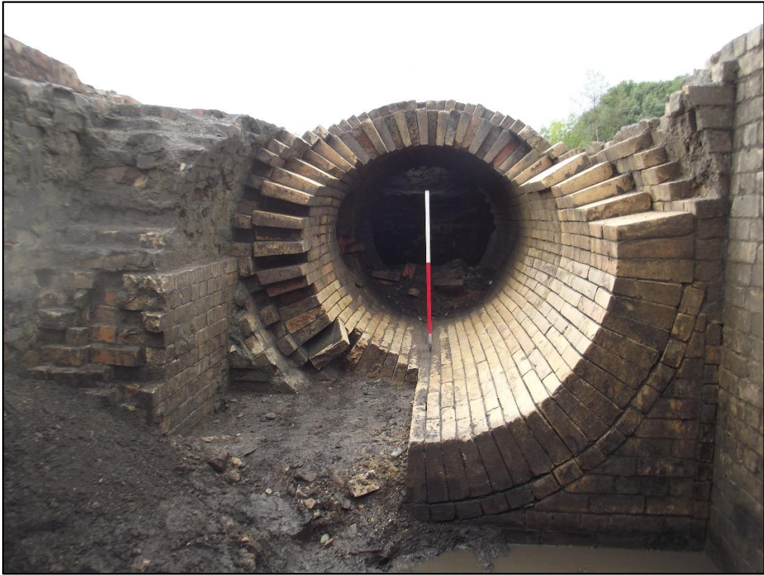
Plate 84. North Coppée Coke oven flue complex, oblique sectional view through damaged main gas flue 2441. Note the method of construction using high quality specialist bricks. Scale is 1m, View to west.
