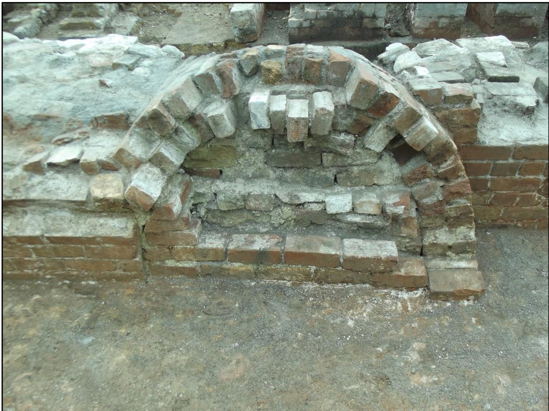
Plate 99. North Coppée coke oven flue complex, Blocked archway 2449. Note brick base group 2468 to the rear of the arch. View to south.
