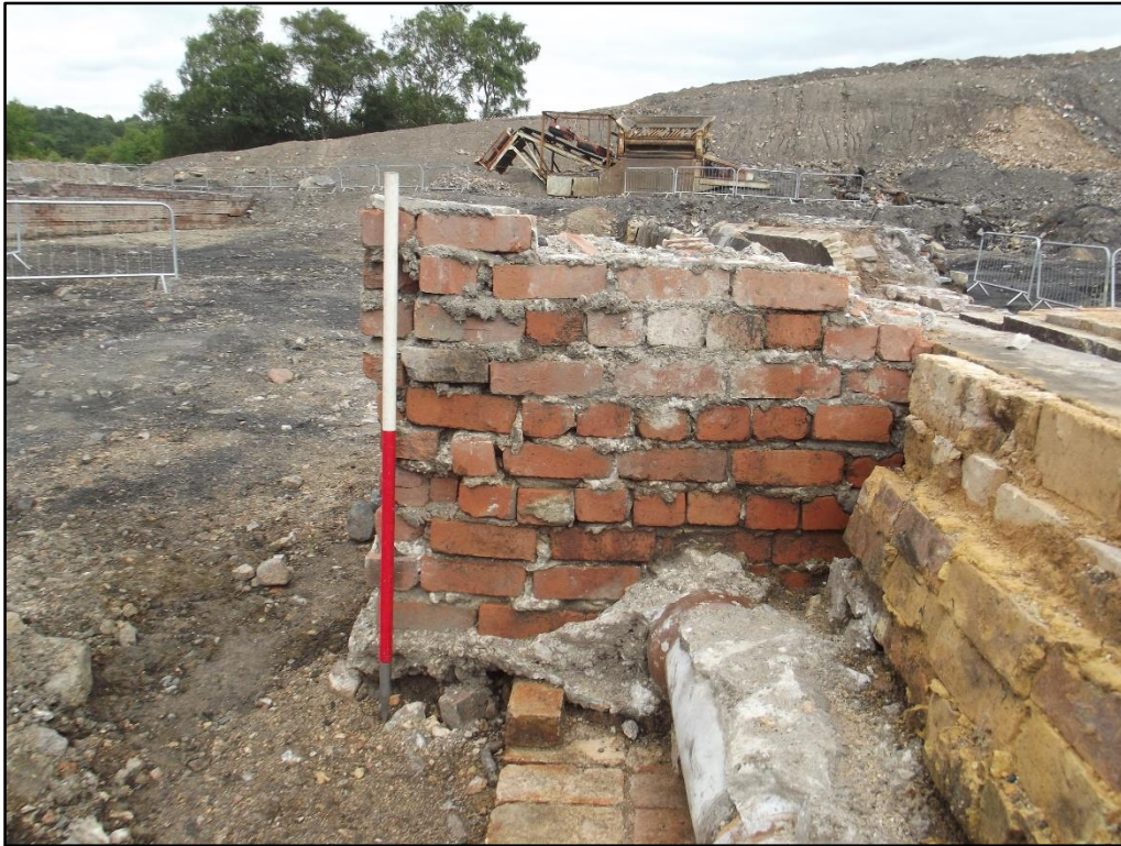
Plate 139. Inspection chamber 2139 cutting the north wall of the main flue for the southern coke ovens. This was almost certainly part of the Thorn Lighting works. View to east.
