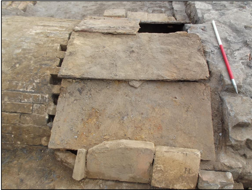
Plate 87. North Coppée coke oven flue complex, iron plates 2444 placed over the uncompleted western terminal of main gas flue 2448 as a removable inspection cover. Note the specialist bricks propping the sheets in place, which were found in their original positions. View to south.
