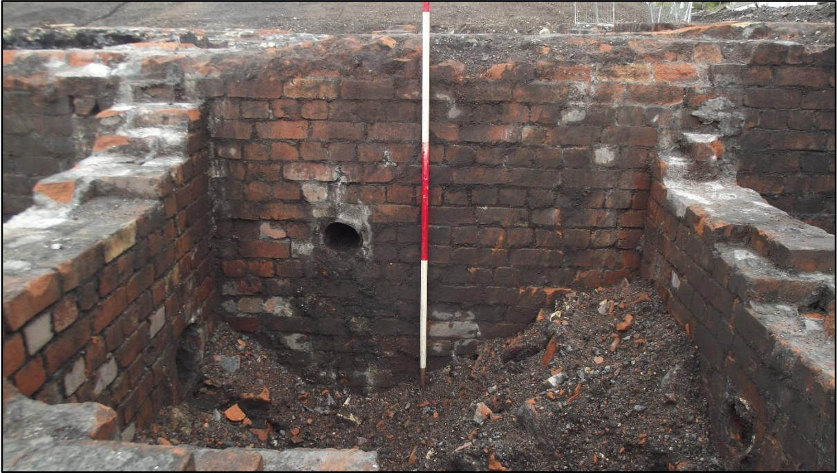
Plate 54. Sheppard washer chamber 2038, view of the interior, looking south. The chamber contained three pipes, the one from elevator pit 2049, and two others, set lower which are likely to have emptied the chamber. The fill of the chamber (2039) was not excavated due to the presence of asbestos.
