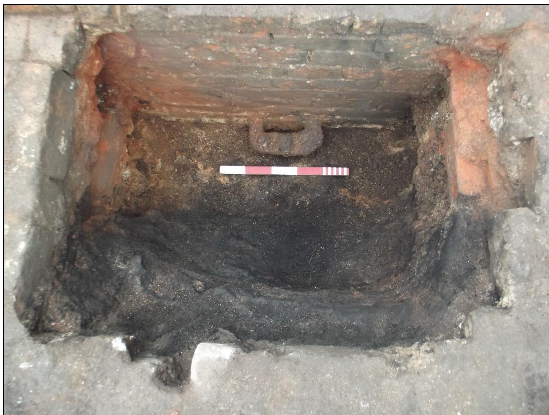
Plate 23. Receiver pit 2361 for part of the Thomas oven door mechanism. Note the iron stay, identical to those on the north side of the ovens.
