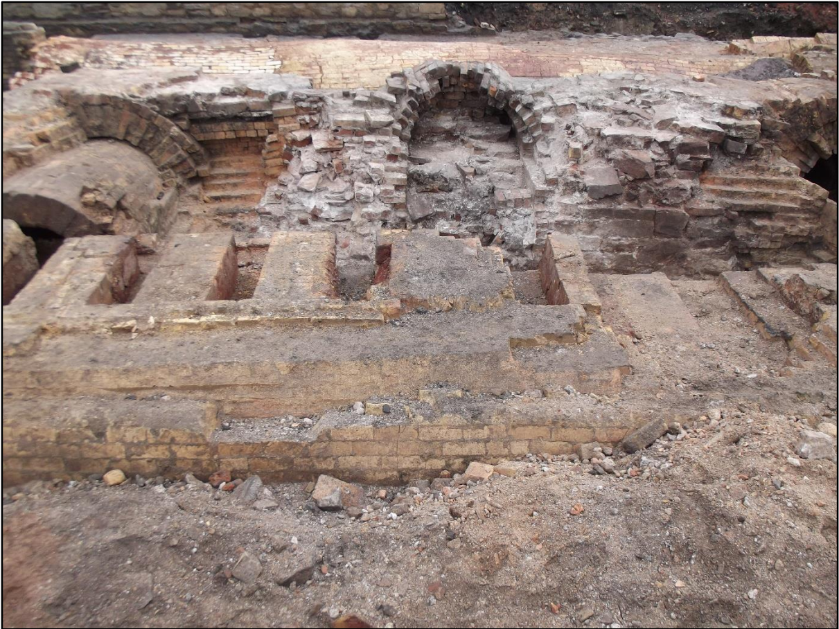
Plate 105. North Coppée oven battery, the mouths of three secondary flues which were open to channel 2480. Note the centre flue (flue 2449) had been blocked during its lifetime. Flue 2448 is on the left and flue 2453 is on the right. View to north.
