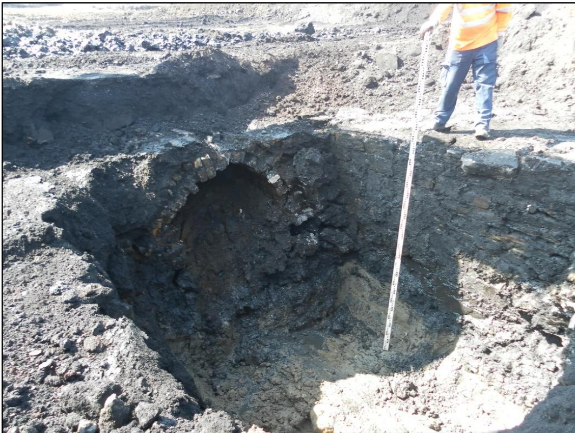
Plate 5. One of the few photographs to show the canal and culvert prior to filling with water. The construction of the culvert can clearly be seen, as can the stone packing (2006) around it. The light brown deposit towards the base may be the natural clay or a build up of silt in the channel prior to construction of the culvert.
