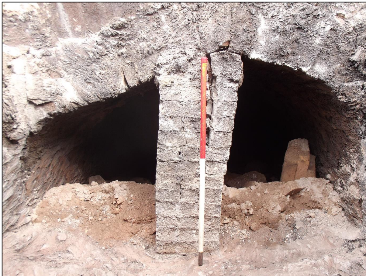
Plate 74. North Coppée oven battery, mouth of the secondary gas flue running from the main gas flue. Note the collapsing arch and the attempt at support being provided by brick pillar 2339. View to north.
