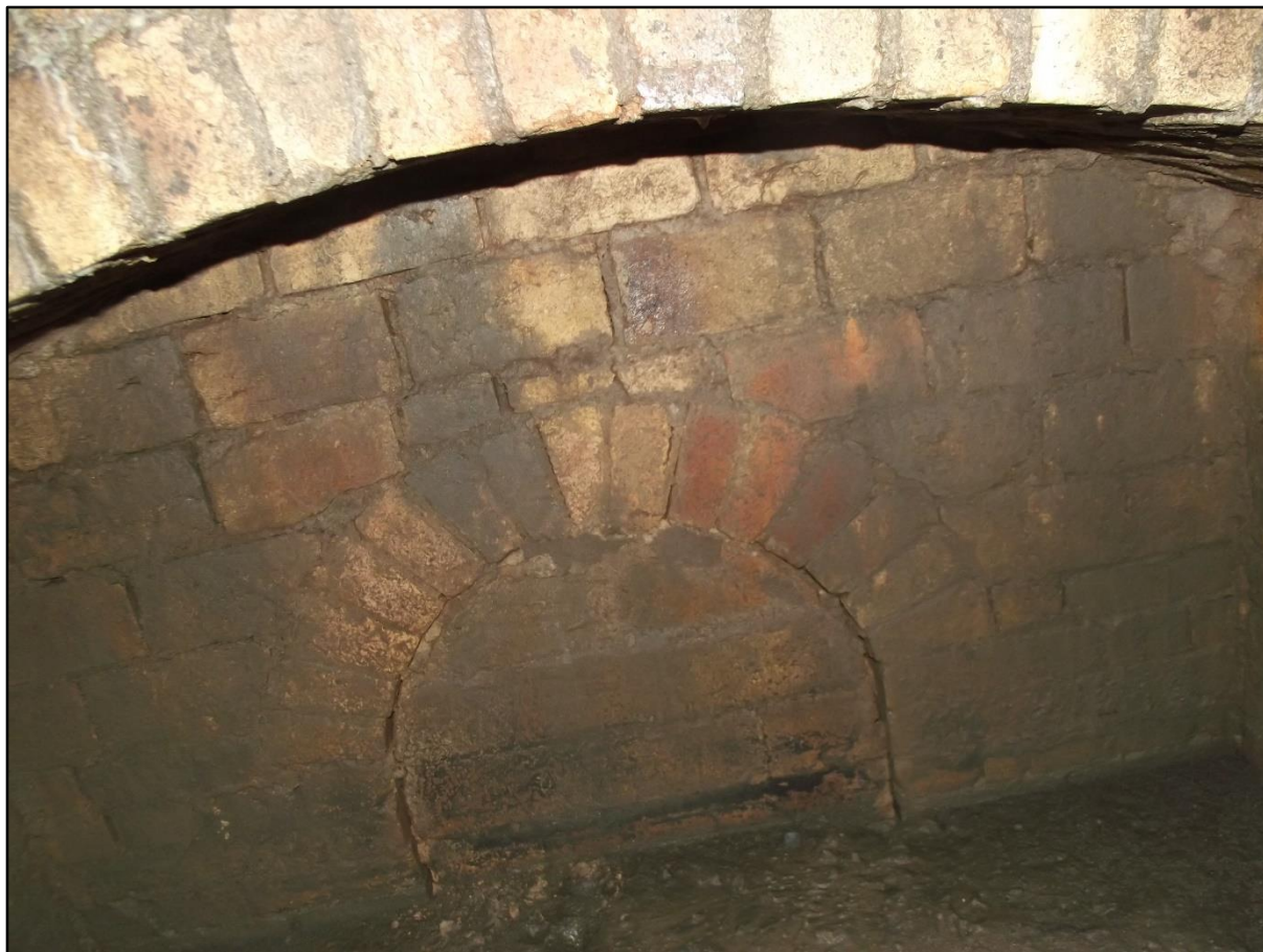
Plate 110. North Coppée coke oven rammer wall, poor photograph of chamber 2485 and blocked flue 2486. Full access to the chamber was not possible for health and safety reasons. View to north.
