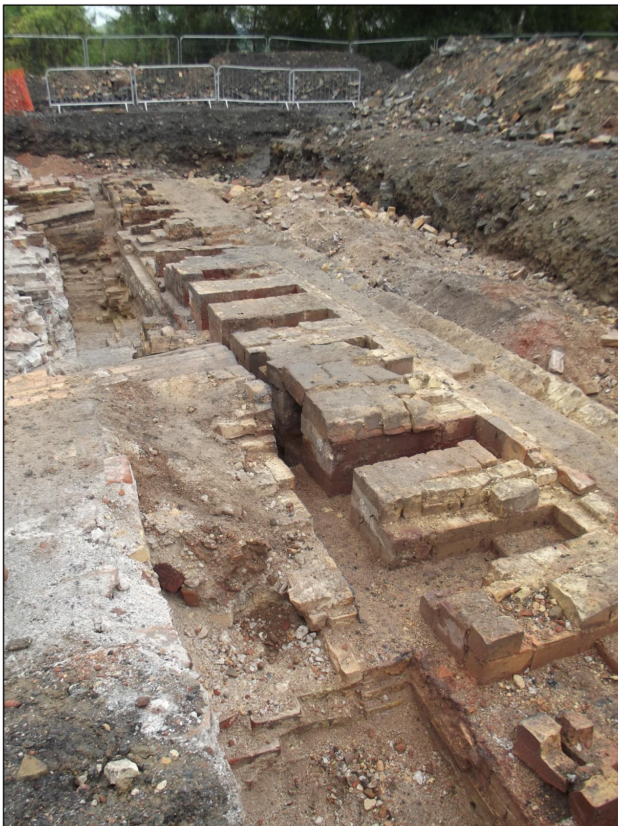
Plate 101. North Coppée coke oven battery, brick built bays group 2468 looking south east
