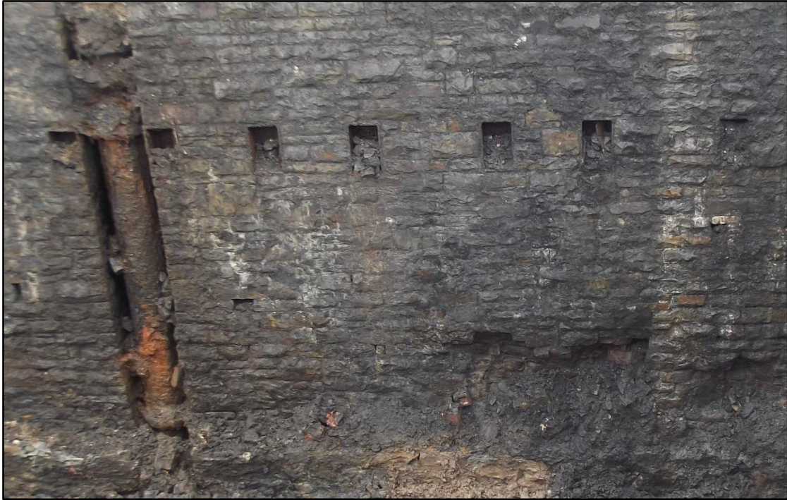
Plate 129. Closer view of the horizontally arranged floor supports in the south wall of the coke bin (2198). View to south
