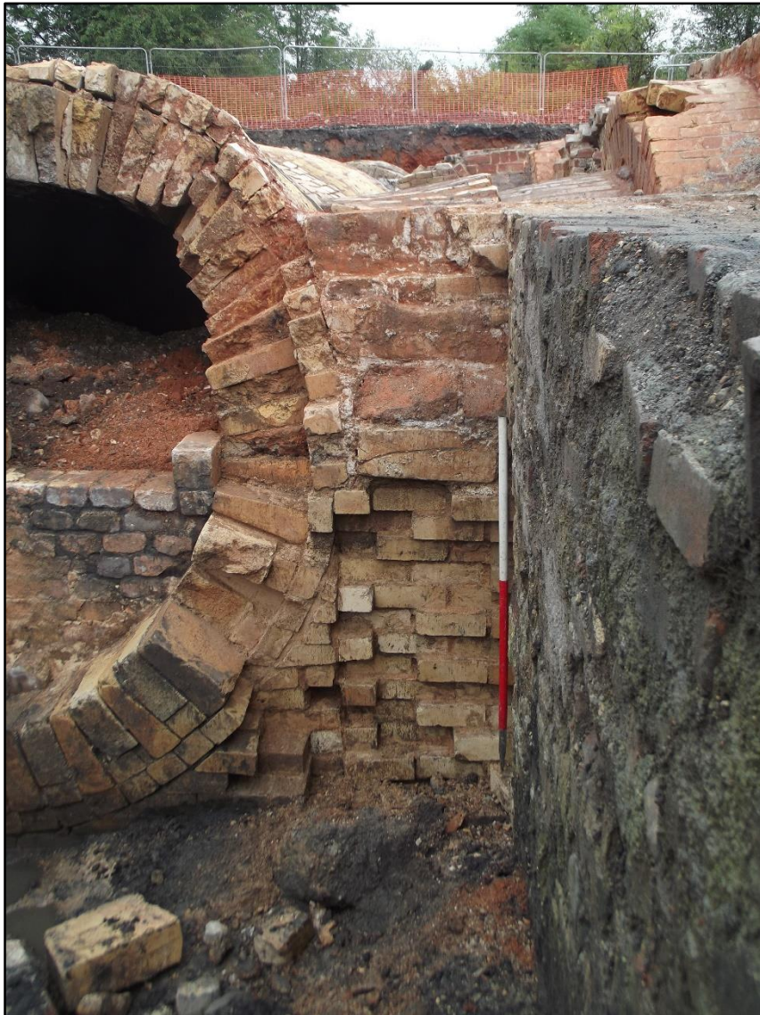
Plate 91. North Coppée coke oven flue complex, mouth of main gas flue 2448 at its junction with chimney base 2132. Floor surface 2439 also served as the south wall of the chamber. View to east.
