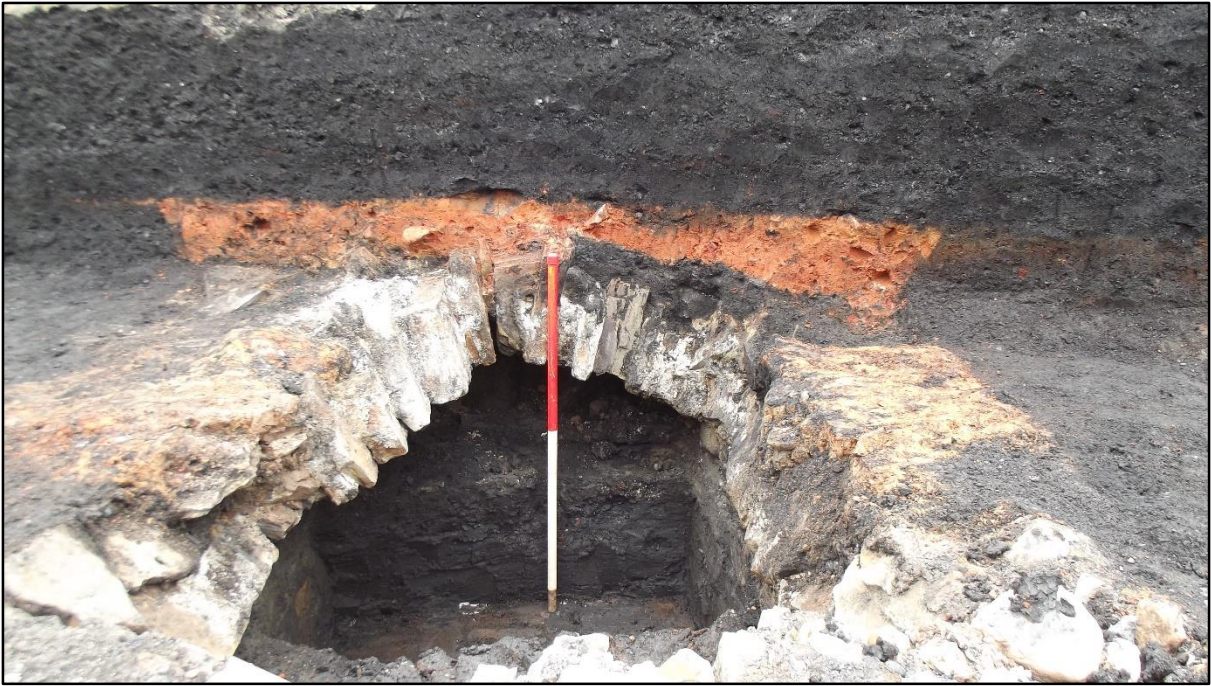
Plate 29. Coke yard area, culvert group 2295 showing the highly distinctive orange clay (deposit 2347) used to seal the culvert. Considerable quantities of coal dust (deposit 2306) must have been present at the time the feature was constructed. View to south.
