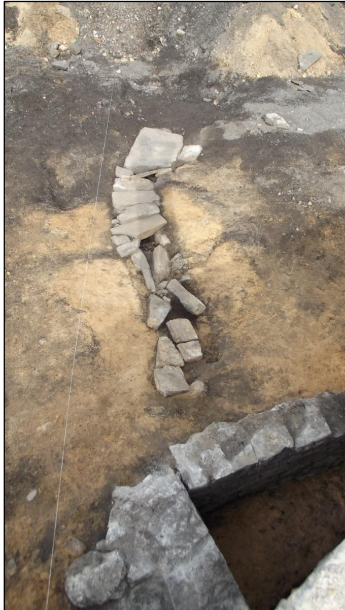
Plate 37. Stone capped drain 2248 may have been cut by the construction of walls 2249 and 2250; the exact nature of the relationship was unclear. This view towards the north east shows the fair faced interior of the structure.
