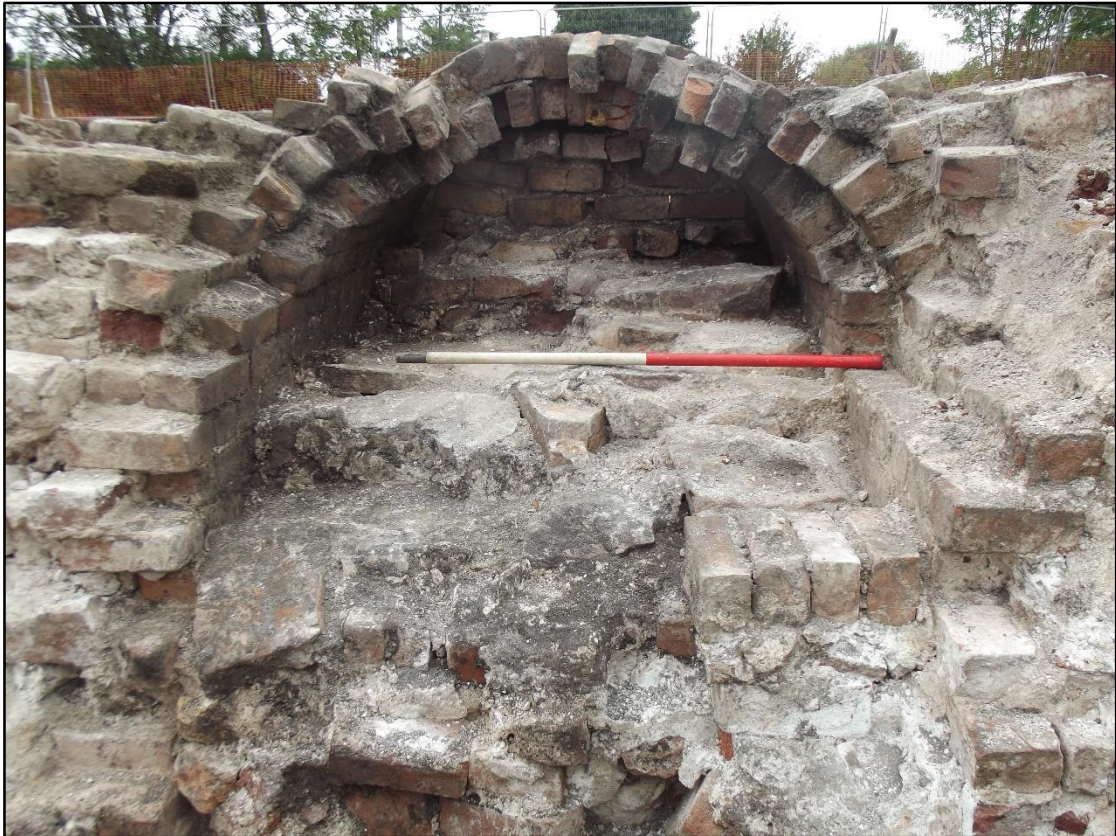
Plate 98. North Coppée coke oven flue complex, rear of blocked archway 2449. This may be a vestigial flue that once connected the main gas flue with brick base group 2468. View to north.
