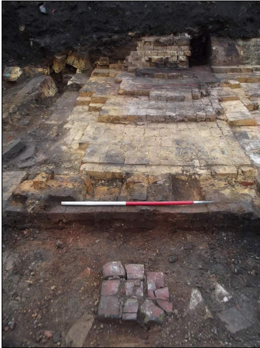
Plate 125. South Coppée coke oven flue complex, another view of the eastern terminus of main gas flue 2012 showing the possible mounting for a grille or similar. View to east.
