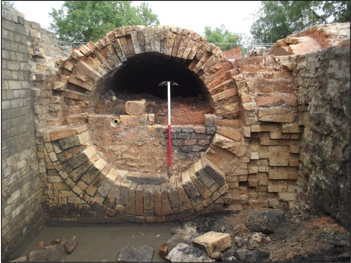
Plate 92. North Coppée coke oven flue complex, partially blocked mouth of the main gas flue within chimney base 2132. This feature was possibly a baffle to reduce the ingress of residue into the chamber base. Note the distortion of the roof, probably caused by heat. View to east.
