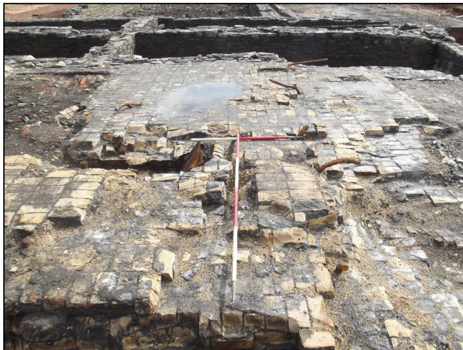
Plate 46. Foundation and mounting pins for the disintegrator and elevator engine. View to north east.
