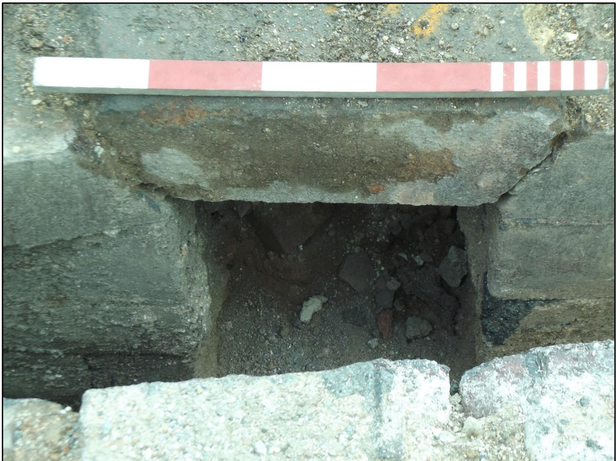
Plate 100. North Coppée oven battery, a capping brick in place over one of the brick bays forming part of group 2468. Note the chamfered nature of the brick to ensure a good seal. Scale is 0.5m
