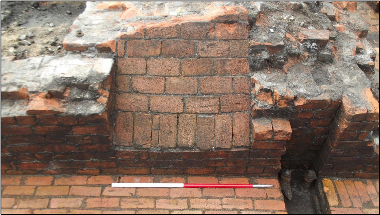
Plate 57. View of chute 2060 in the north passageway. Note the recess in the wall to the right of the chute to allow for insertion of a timber sleeper. Scale is 1m.
