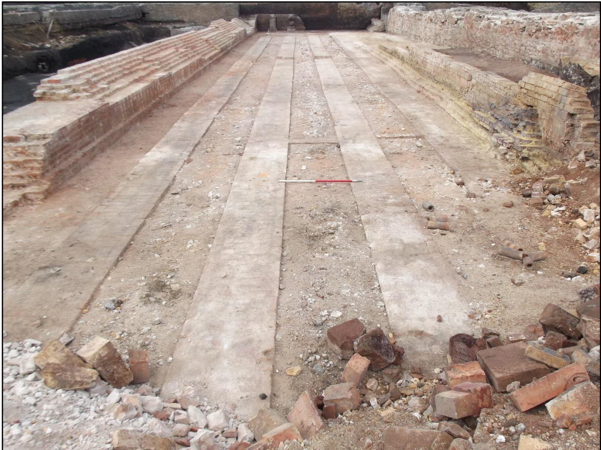
Plate 68. North coke oven battery, strip foundations 2328 (left) to 2331 (right). Retaining wall 2341 is on the far left of the image whilst the remains of the main heat flue are on the far right.
