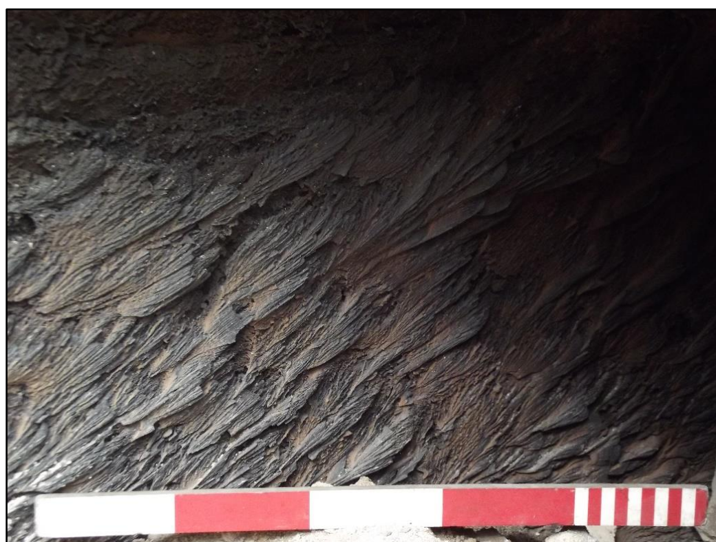
Plate 76. North Coppée coke oven battery, characteristic flow lines in the residue left on the side walls of the secondary gas flue. Scale is 0.5m.
