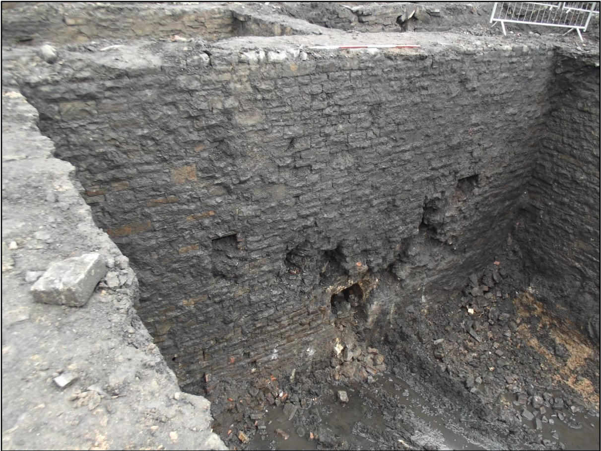
Plate 130. View of the west wall of the coke bin (2181) showing the damaged recess that was probably part of the transport system for moving the coke from the bin to the furnace tops. View to north west
