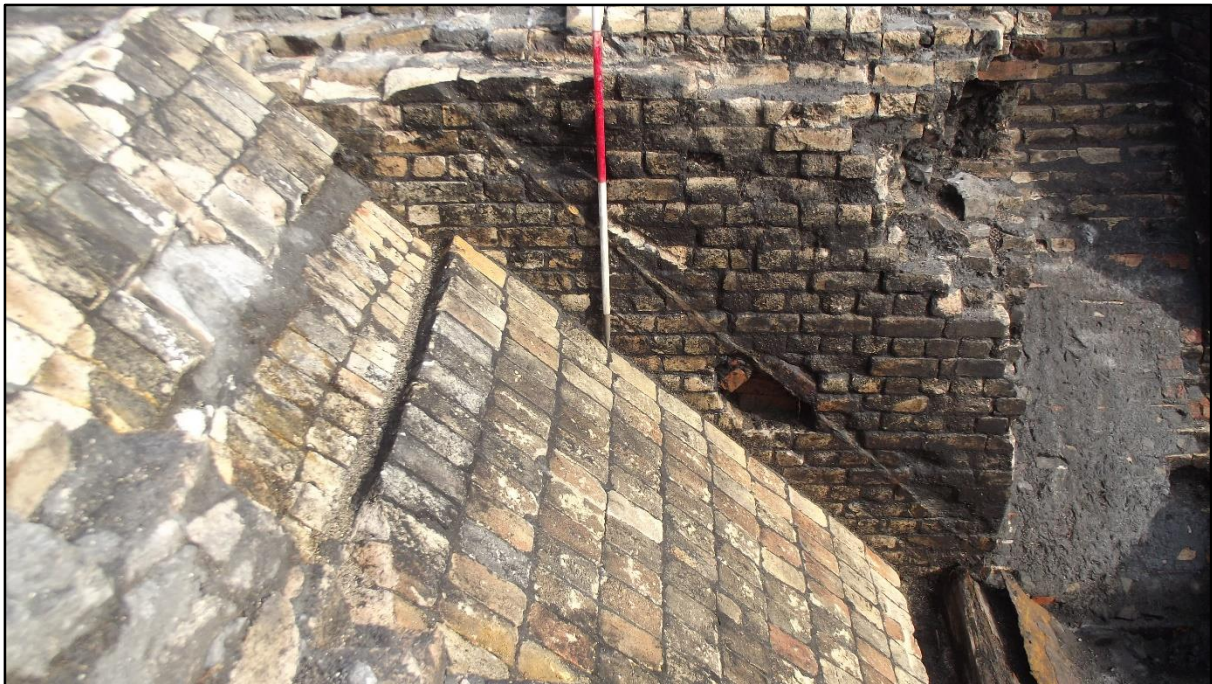
Plate 42. The western elevator chute 2063 for the Carr's disintegrator. Note the parallel lines on the far wall marking the position of the iron sheets that formed the actual wearing surface of the elevator. This sheeting was intact at a lower level, as seen at the bottom right of the photograph. View to north.
