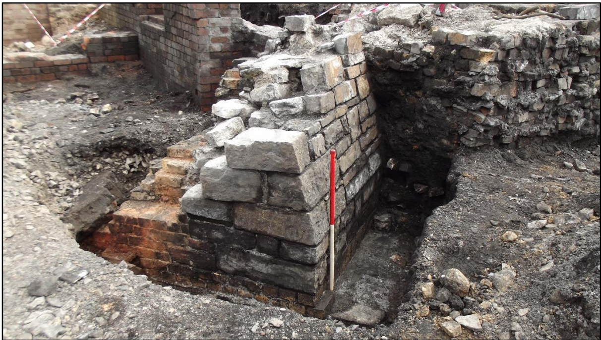
Plate 19. Battered gable end of the surviving element of the Thomas ovens. Note excellent quality of the dressed stonework.
