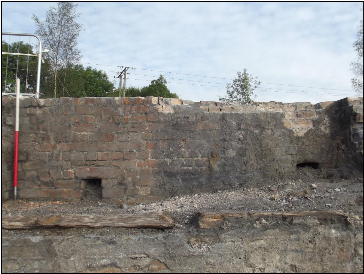
Plate 107. North Coppée coke rammer wall, alcove 2321 showing the remains of timber planking and two recesses in the south elevation of wall 2324. View to north.
