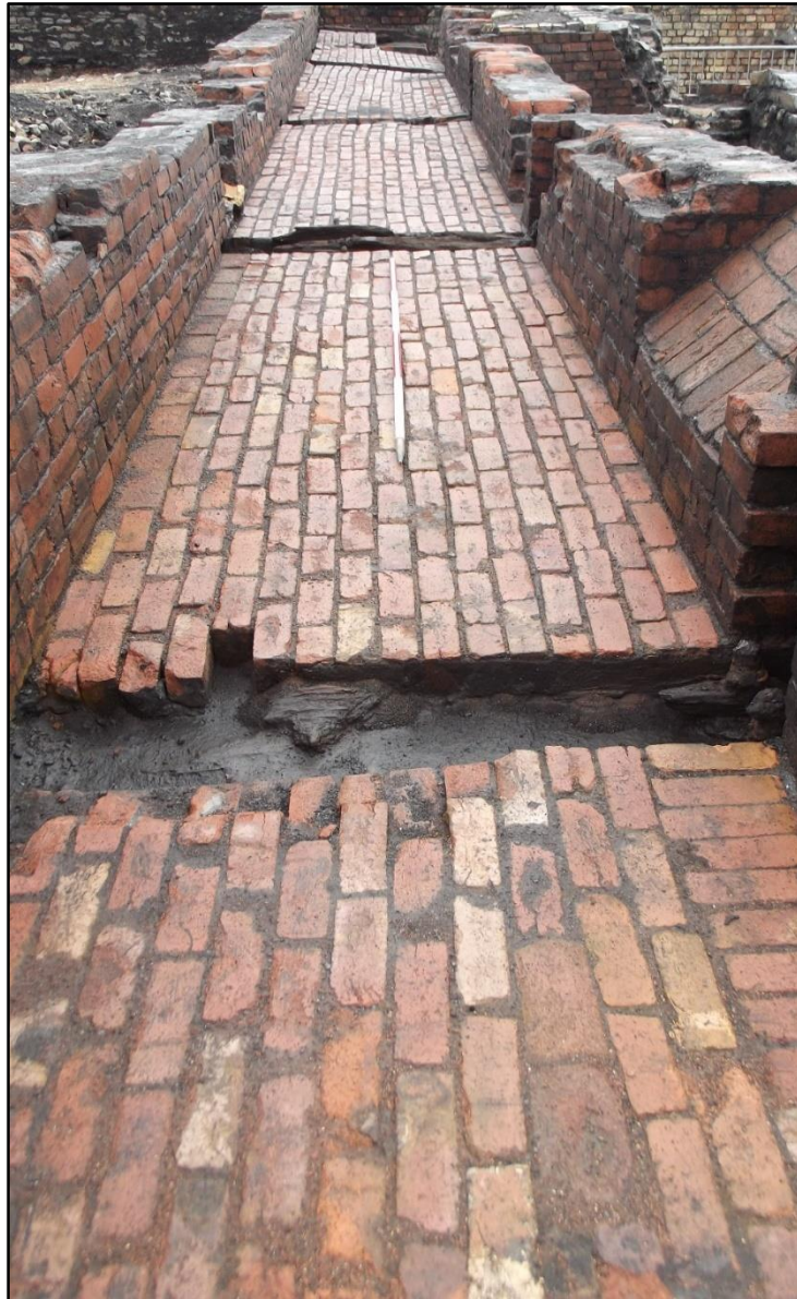
Plate 56. The north passage of Group 2059 (brick floor 2072) showing chute 2060 to the right. Note the sleeper locations and the slots built into the flanking walls that would have permitted easier replacement of the sleepers. Note how the pins are off-set to the right (south) side of the passage, possibly to allow limited access to the screw conveyor for clearing blockages and repairing the machinery (see also Plate 59). View to east.
