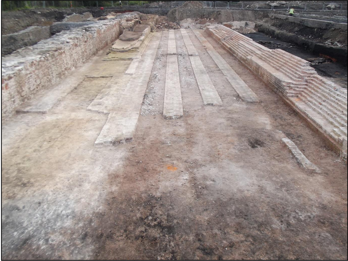
Plate 67. Remains of the strip foundations of the north battery of Coppée coke ovens. View to east. Wall 2314 is visible to the right of the photograph whilst wall 2324 is visible on the left. The space between is filled with a series of linear brick foundations, and the base of a single, large flue (2340 and 2343) is located adjacent to the left hand wall. View to north east.
