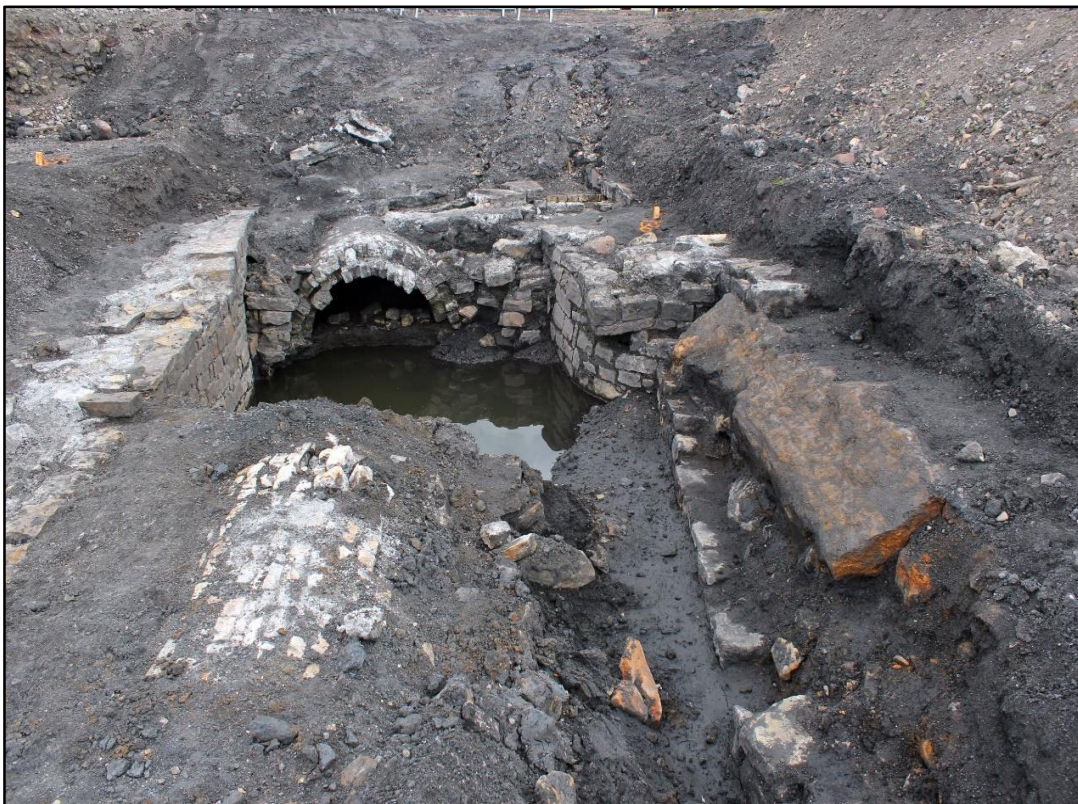
Plate 4. Anthony Bacon's canal. The orange/brown ramp on the right of the photo is believed to be a lading and unlading ramp, to aid transfer of materials to and from the tub boats. Note also the curved walling to allow the widening of the canal for the passage of boats. Note the later brick culvert built into the canal. View to east.
