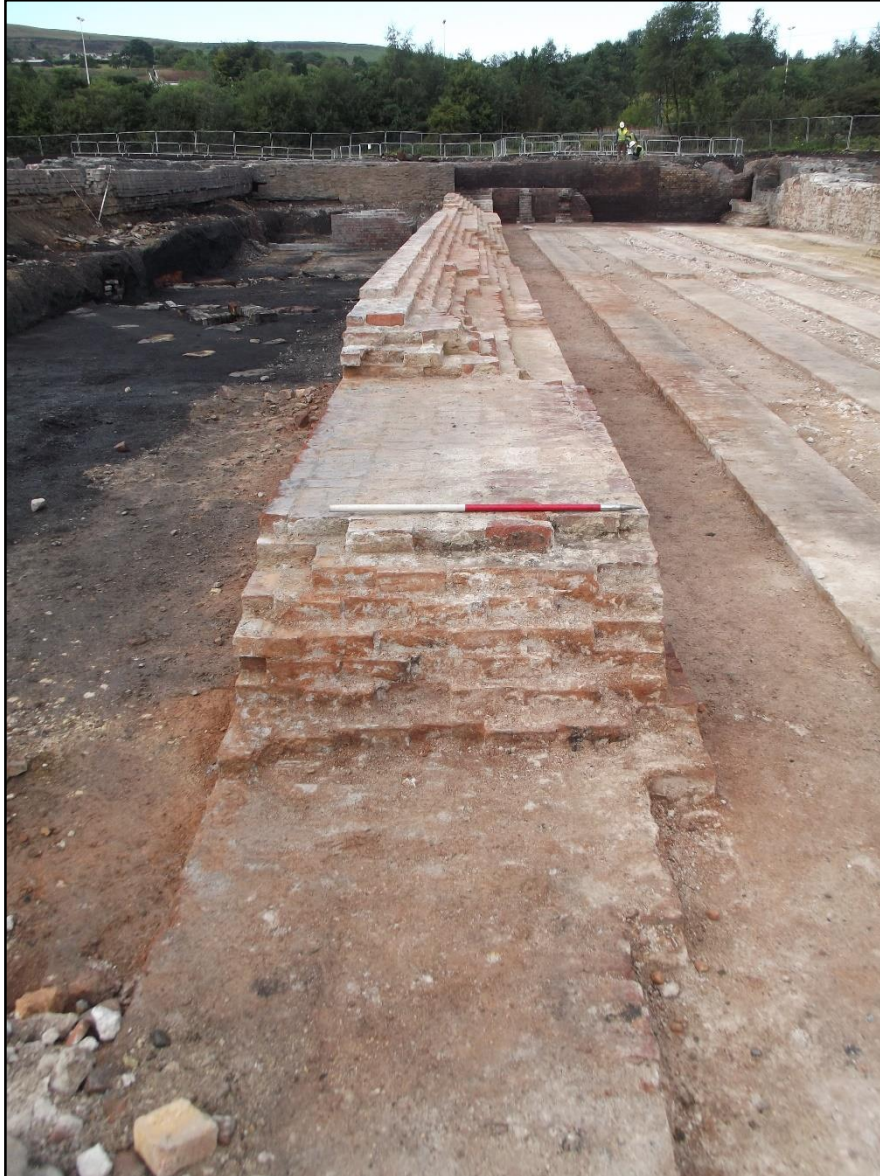
Plate 69. North Coppée coke oven battery, retaining wall 2314 looking along its length. View to west. The vertical left hand face of the wall is likely to mark the location of the front of the Coppée ovens.
