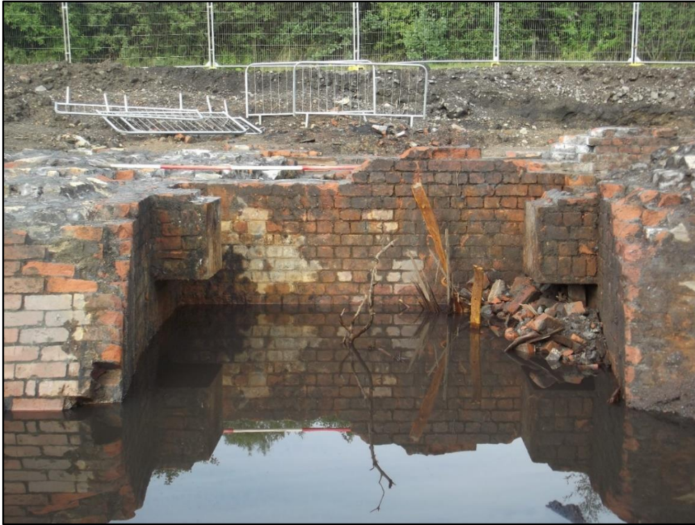
Plate 50. Recess in hopper 2055 showing the iron and brick wall supports on either side. View to west.
