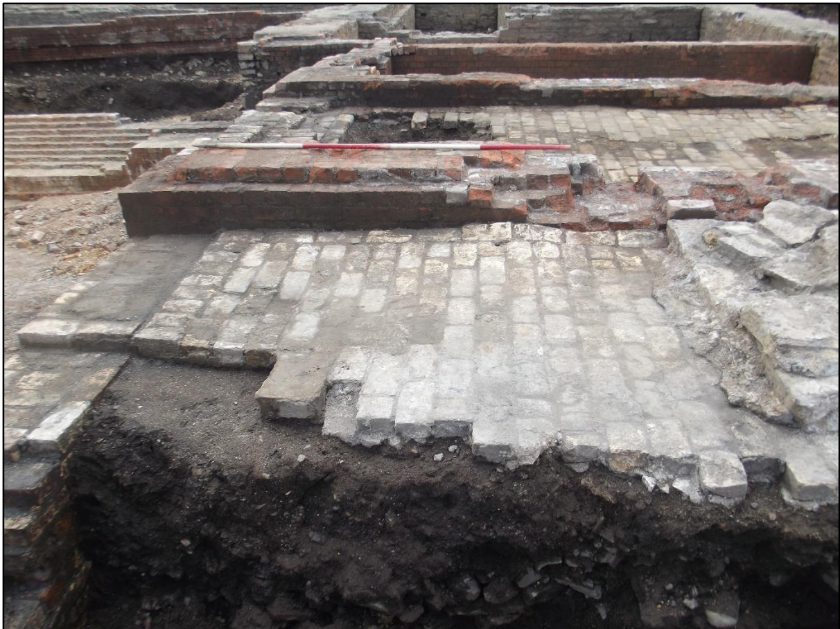
Plate 65. North Coppée coke oven battery, floor surface 2221 showing the cut for the modern pipe run (2228). Floor 2221 was almost certainly related to the transportation system for moving coal to the top of the coke ovens but the insertion of the masonry partition (wall 2229 on the right of the photograph) would have significantly affected the space available.
