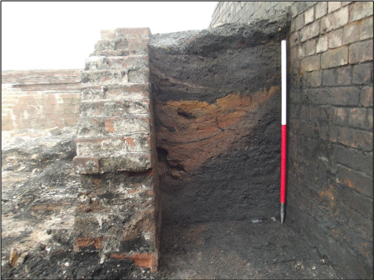
Plate 62. North Coppée oven battery. Insulation deposit 2313 sandwiched between the western end of the north coke oven battery (wall 2315 on the left) and the coal storage bunker (wall 2215 on right). Note the deposit has been heat affected. View to south.
