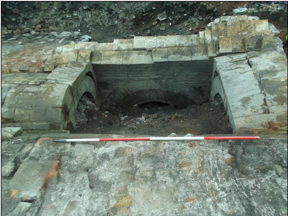
Plate 93. North Coppée coke oven flue complex, brick chamber 2464, which was the junction of flues 2456, 2448 and 2459. Scale is 2m, View to north.
