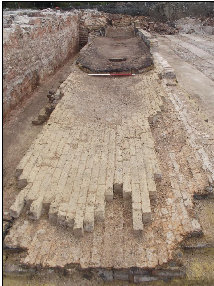
Plate 70. Northern Coppée coke oven battery, surviving floor (2340) of the main gas flue. Note the highly vitrified original floor of the flue just above the ranging rod. View to east.
