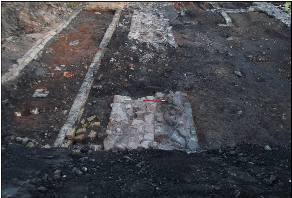
Plate 126. South Coppée coke oven flue complex, exposed remains of the north coke rammer wall (wall elements 2537, 2570, 2533 and 2534). The double skinned nature of the masonry is evident, as is the later wedge shaped cut (cut2530) through the wall, associated with either construction or demolition of the Thorn Lighting works. View to east.
