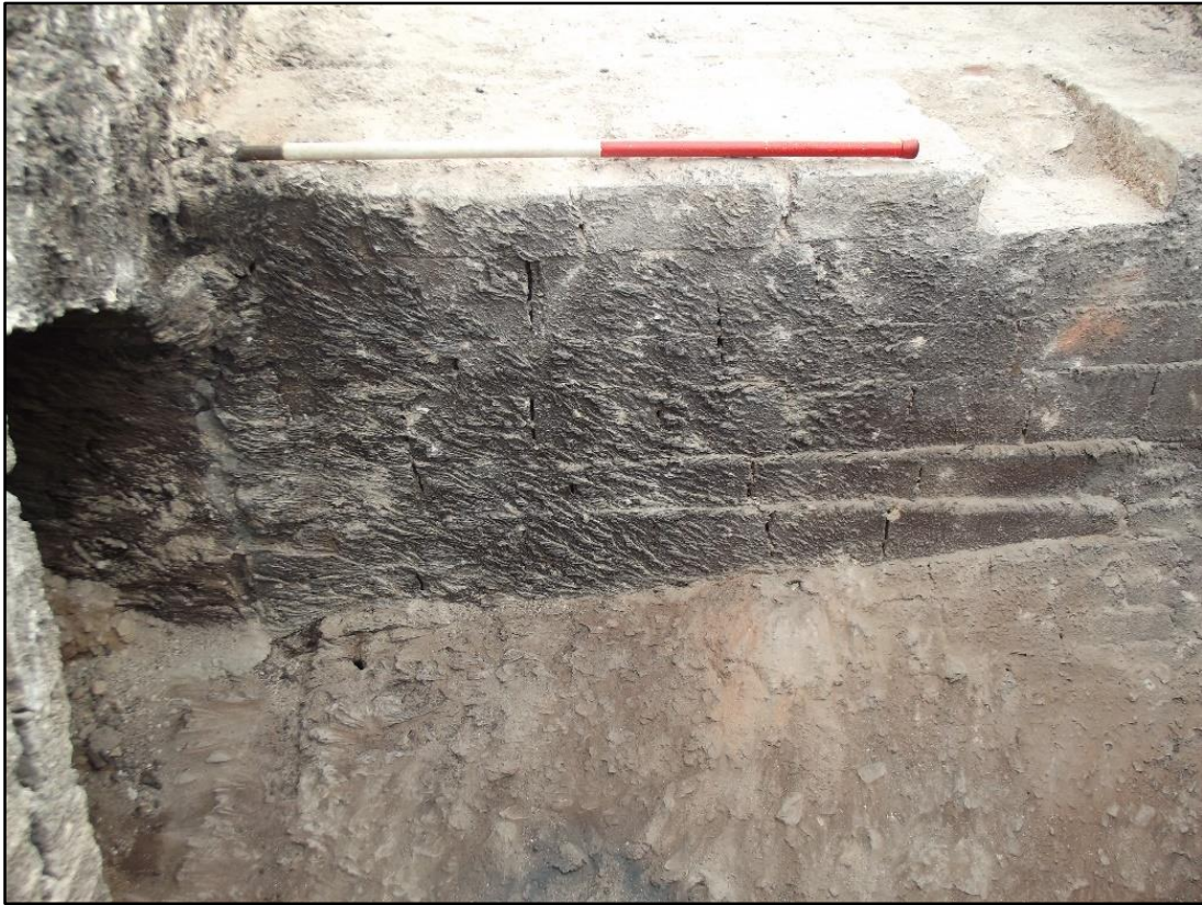
Plate 73. North Coppée oven battery, secondary gas flue chamber 2338. The floor of this chamber sloped in two dimensions, demonstrating the highly skilled nature of the workmanship involved. Note the extensive vitrification. View to east.
