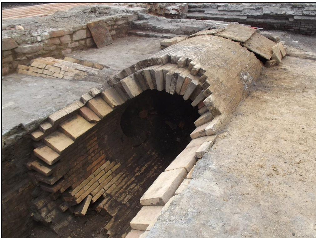
Plate 88. North Coppée coke oven flue complex, oblique view of the western terminal of main gas flue 2448. Several interesting features are visible including the mouth of secondary flue 2442 inside the main flue, and iron plates 2444. View to south west.
