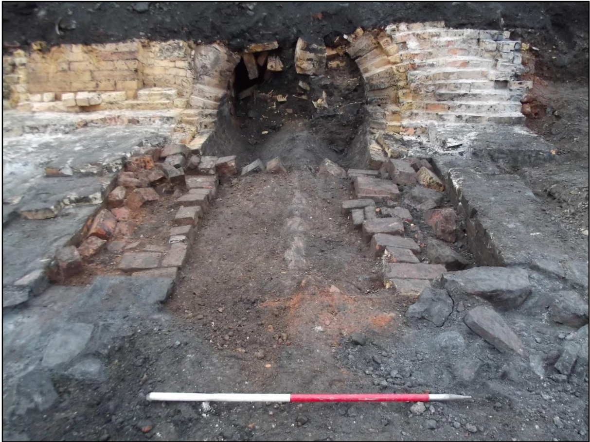
Plate 124. South Coppée coke oven flue complex, view of secondary gas flue 2526 and chimney base 2509. Note the ridge of accreted material in the centre of the channel and the deliberate attempt to narrow the chimney base chamber. View to east.
