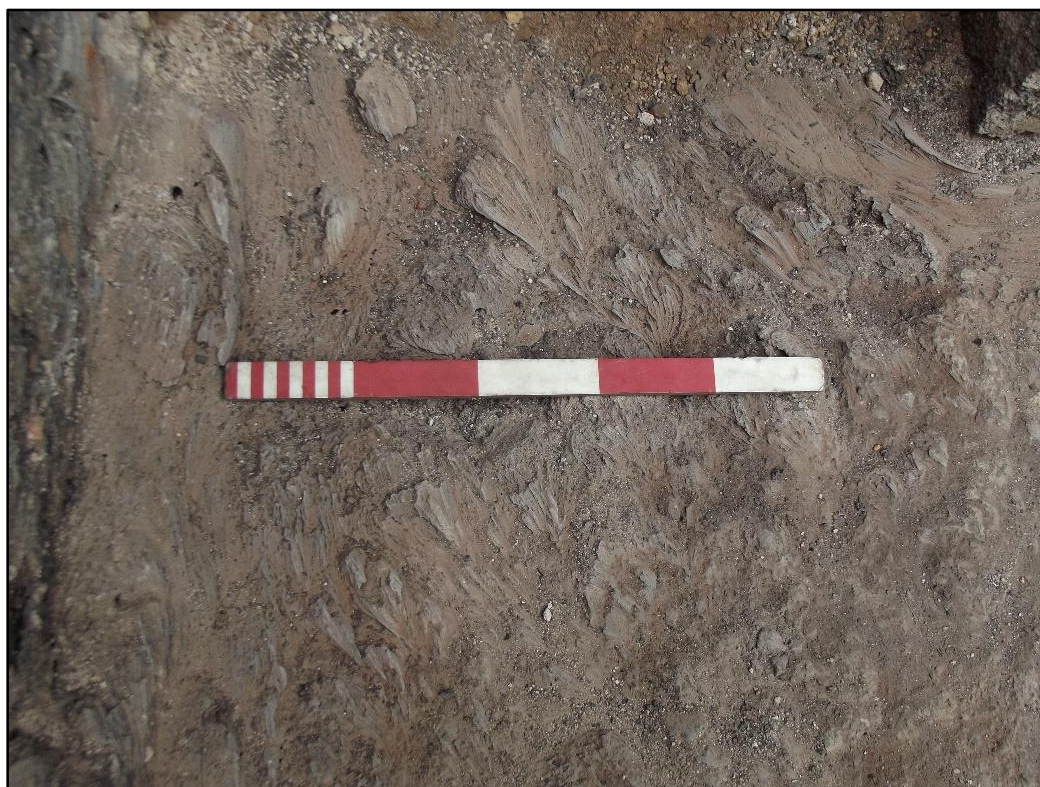
Plate 75. North Coppée oven battery, flow lines in the residue within secondary gas flue 2338. Scale is 0.5m
