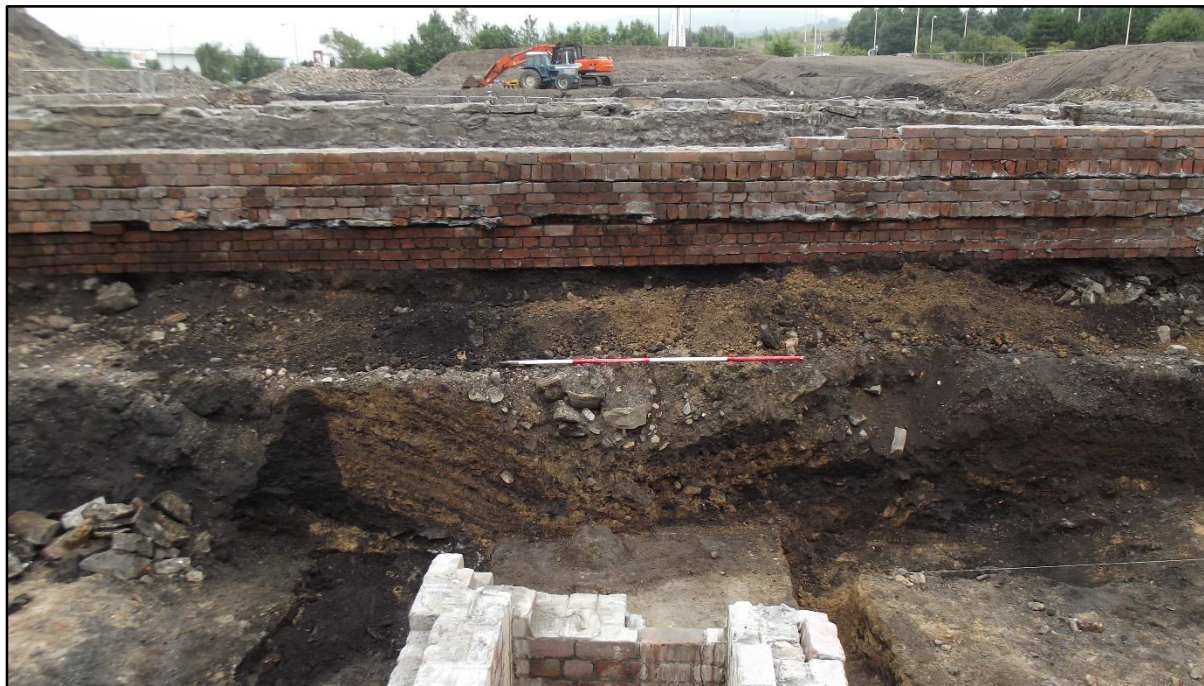
Plate 134. North Coppée coke oven coke bench, cut for modern brick chamber 2309.
