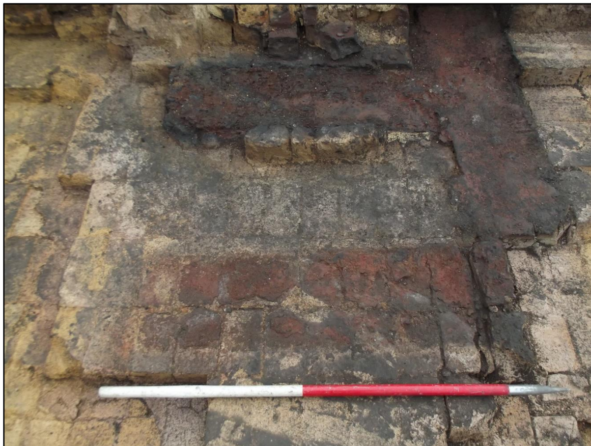
Plate 122. Southern Coppée coke oven flue complex, remains of recesses 2560 (closest) and 2559 visible as heavily vitrified areas of brick. View to east.
