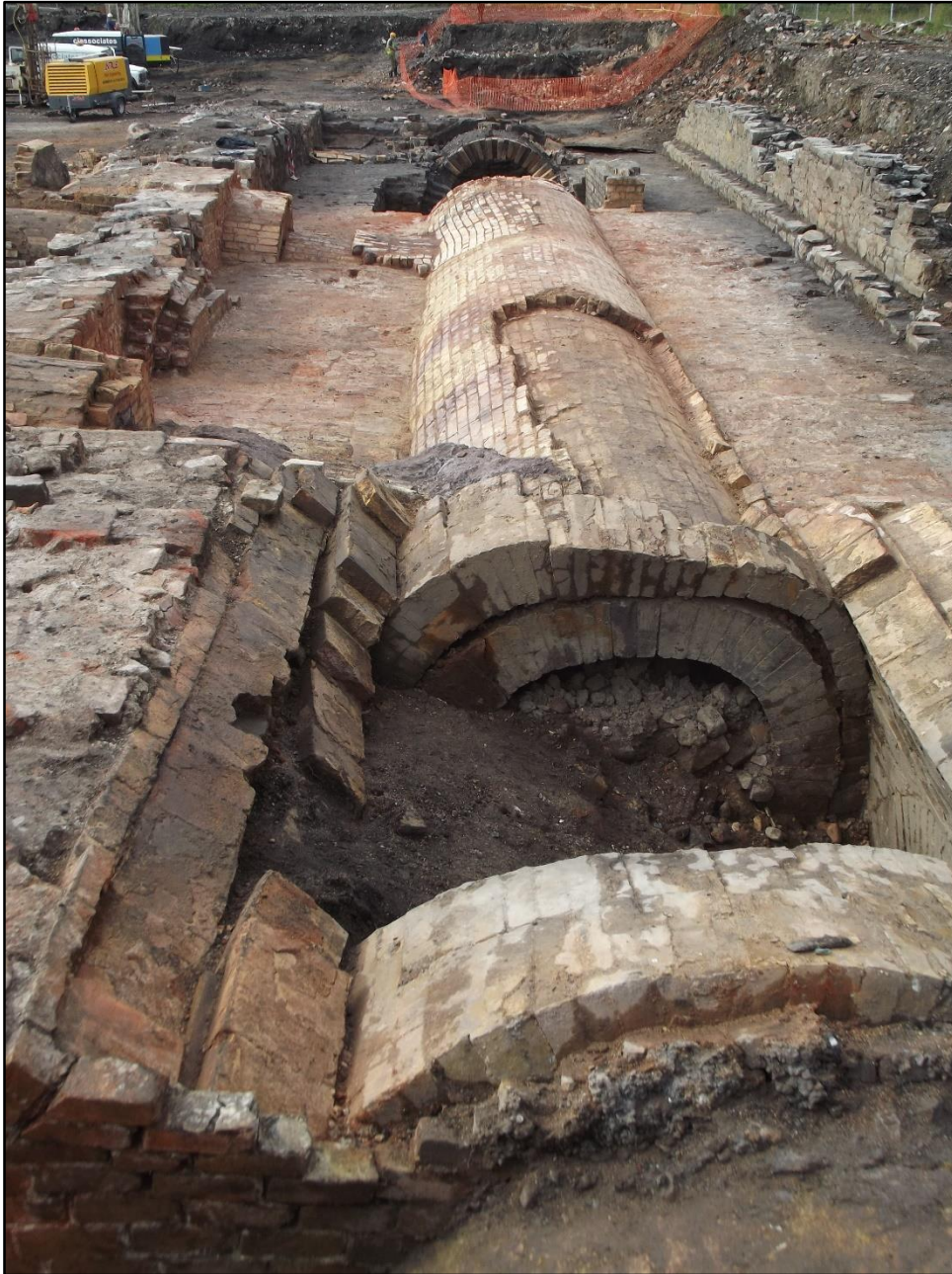
Plate 82. North Coppée coke oven flue complex, showing the arrangement of walls and floors to create a substantial 'cradle' in which to construct main gas flue 2448. Junction base 2464 is closest to the camera. View to west.
