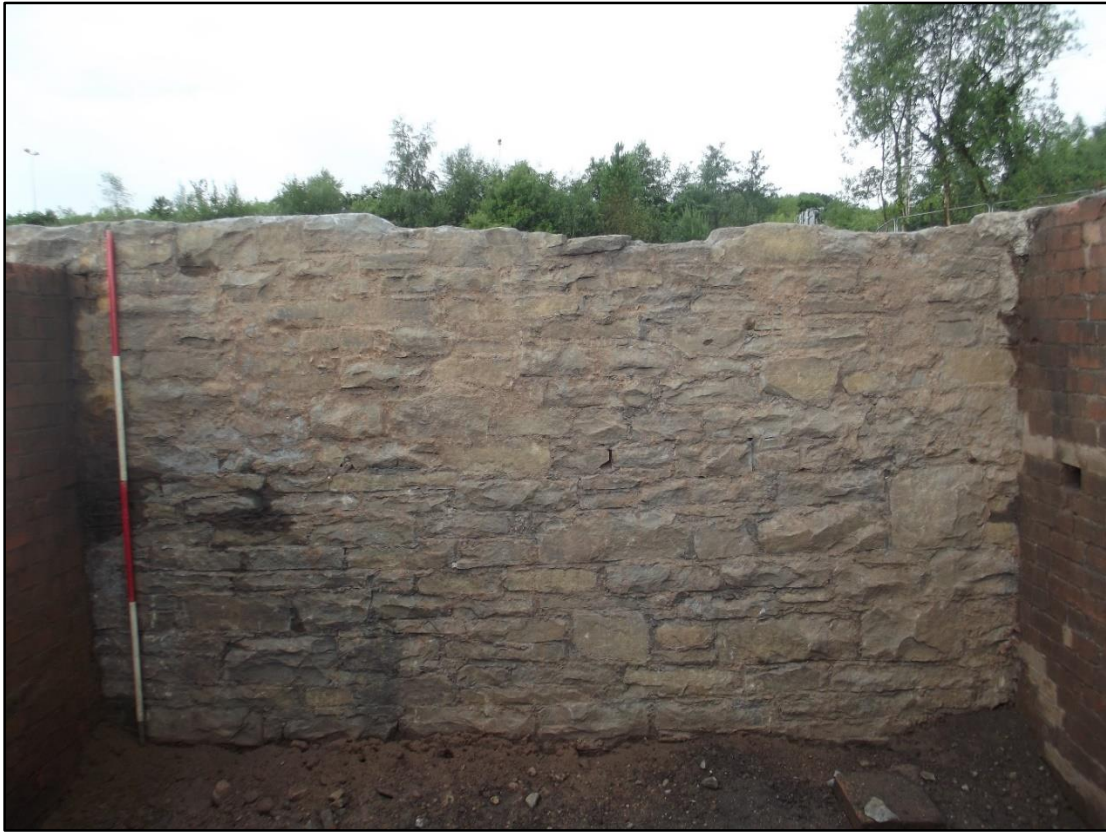
Plate 61. Phase 3b coal storage bunker. View of the eastern (internal) elevation of wall 2213. Brick partition walls 2217 (left) and 2218 (right) are also visible. Scale divisions are 0.5m.
