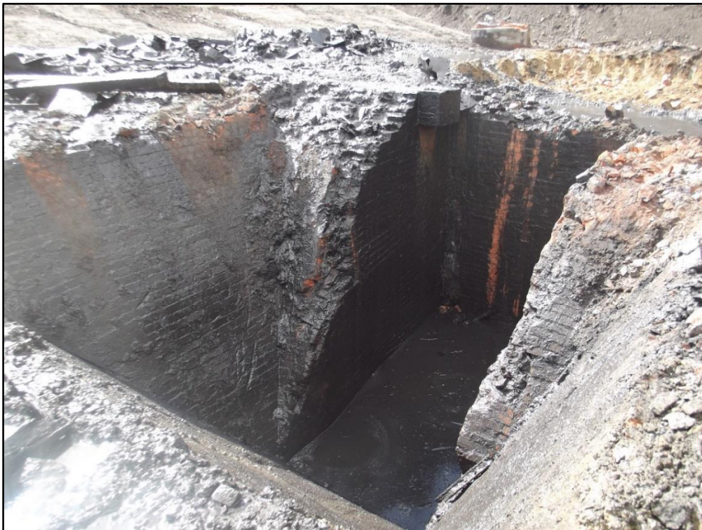
Plate 51. Hopper 2055 following clearance of the water and debris that it had contained. This feature is exactly as depicted in a drawing contained in The Engineer of 12th December 1895. The rectangular chamber housed part of the chain bucket system.
