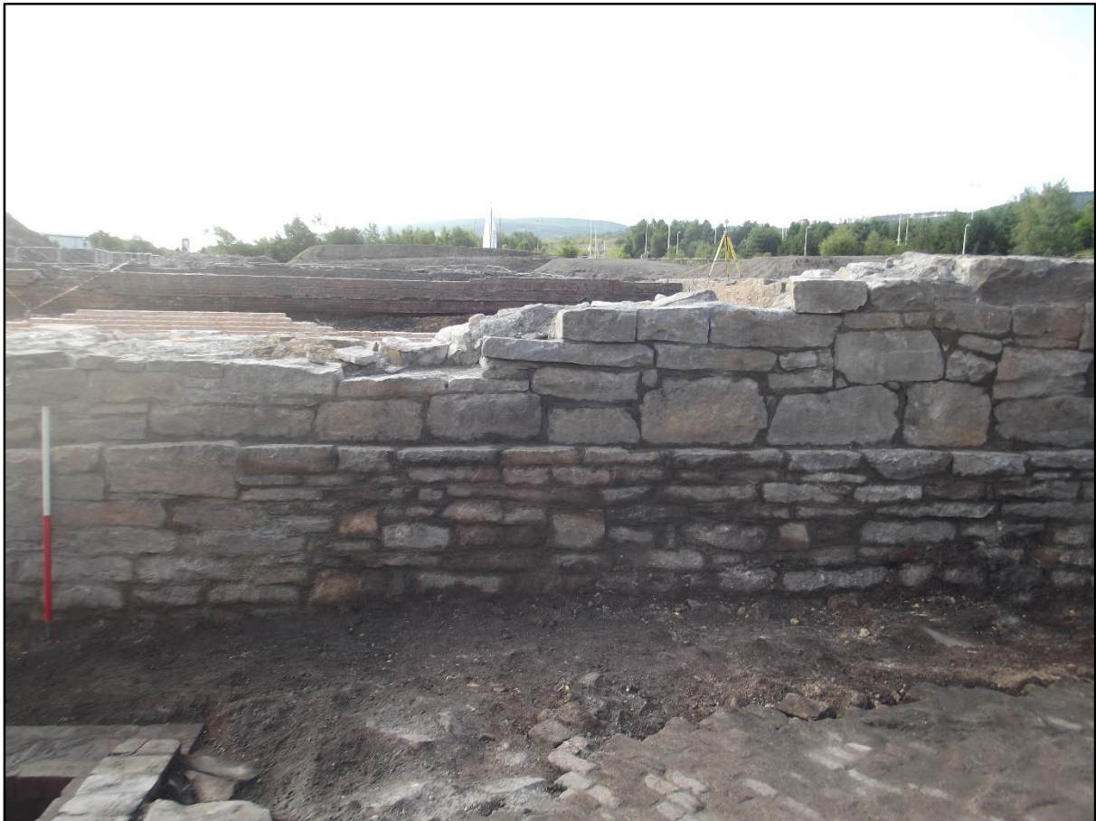
Plate 106. North Coppée coke oven rammer wall, north elevation of wall 2324 showing constructional differences. View to south.
