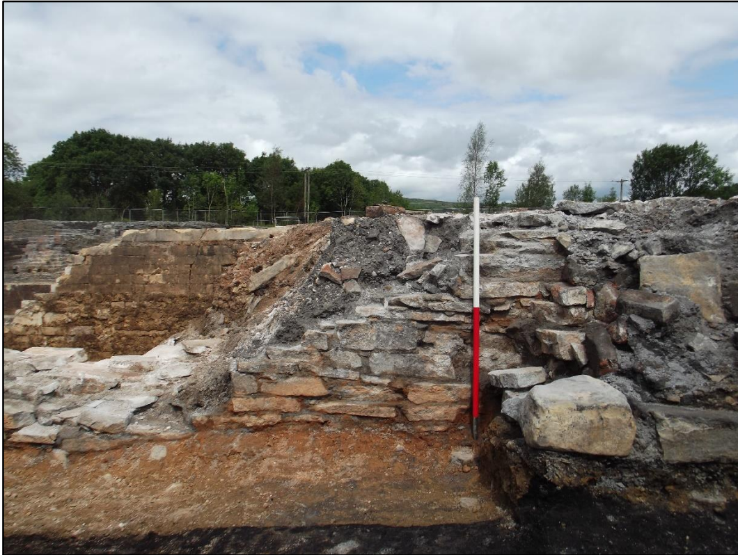
Plate 117. South Coppée coke oven battery, useful photograph showing the south elevation of the south main gas flue (flue 2012 at the rear left, and coke rammer masonry walls 2009 (centre) and 2133 (right). The very straight construction cut for the wall (cut 2135) is clearly visible at the bottom of the photograph. View to north.
