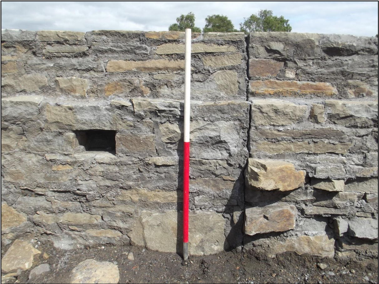
Plate 48. Phase 3a coal storage bunker group 2172. Abutment of walls 2176 (left) and 2181 (right). View to east. The slot (recess 2192) in wall 2176 is believed to be a beam slot to support a floor level, working in conjunction with the step in the walls visible in the photograph.
